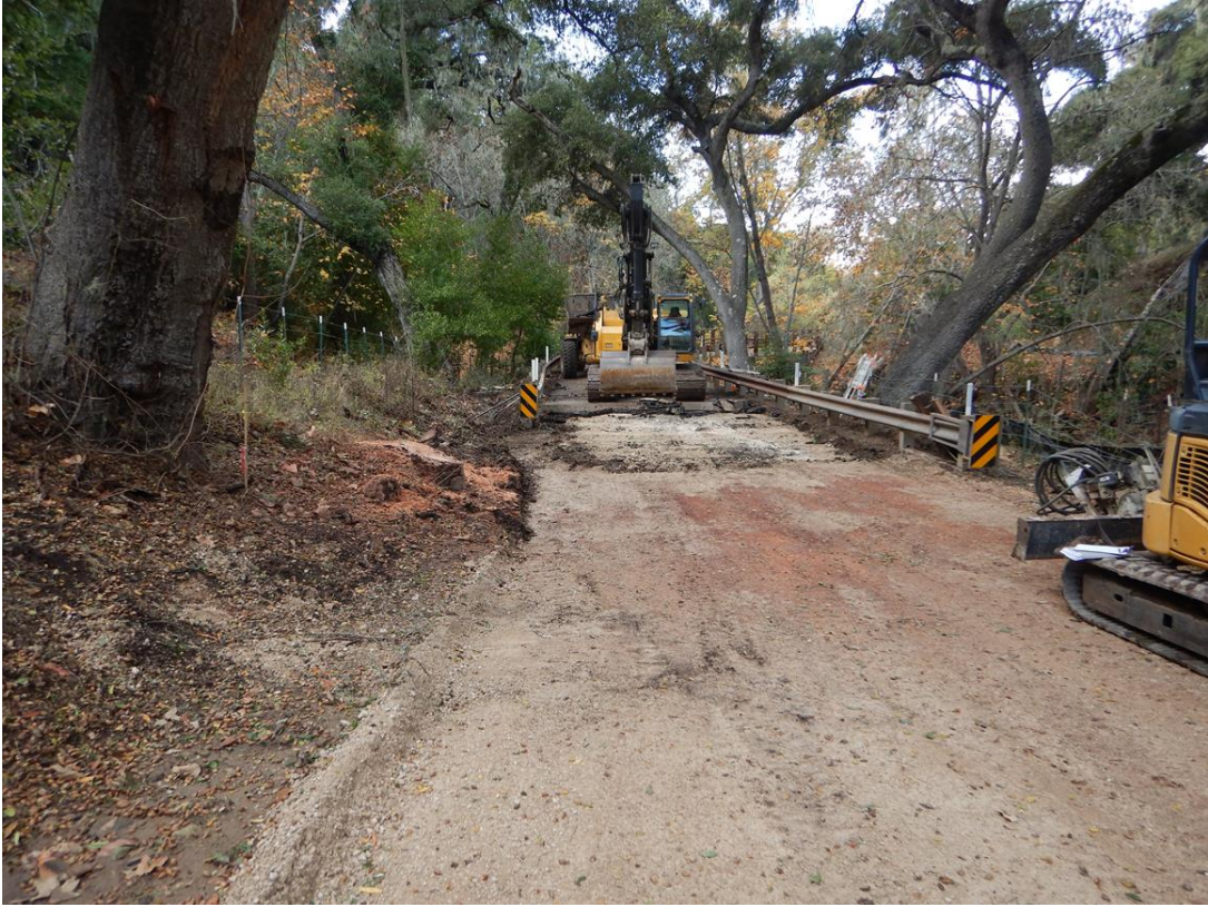
Figure 8: Asphalt removal after the guardrail was moved and the tree removed.
