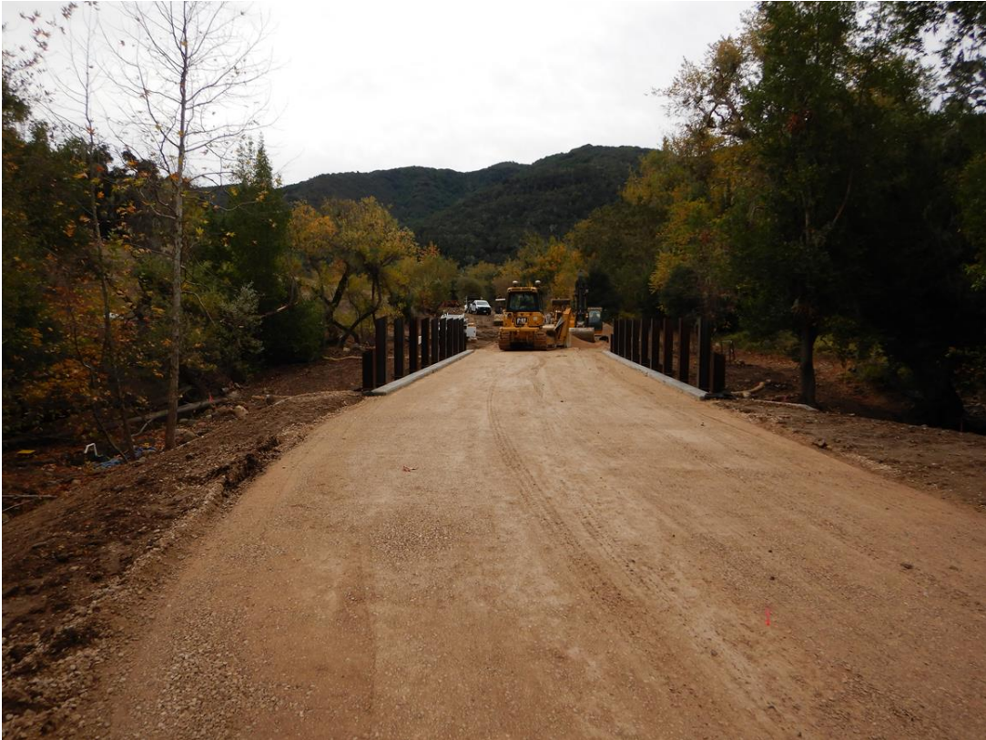
Figure 5: Installing road shoulders and road base
