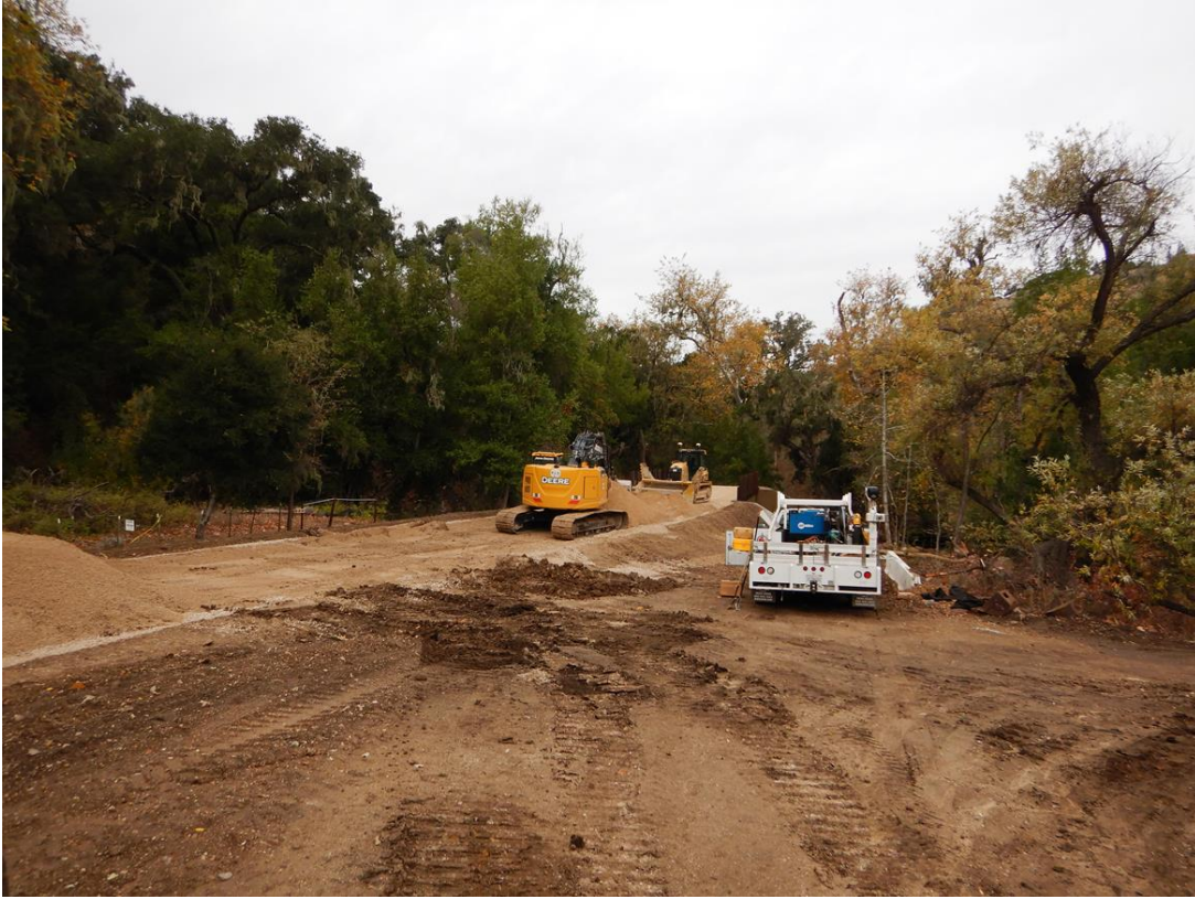
Figure 4: Installing road shoulders and road base.
