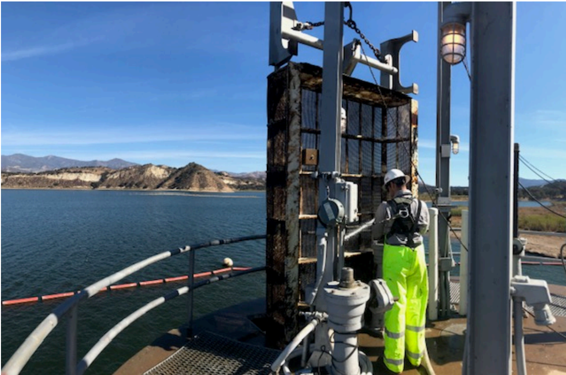
Cleaning fish screens and exercising slide gates at the North Portal Intake Tower
