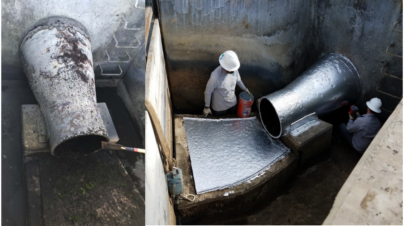
Cleaning and coating Lauro Reservoir inlet pipeline in energy dissipation structure
