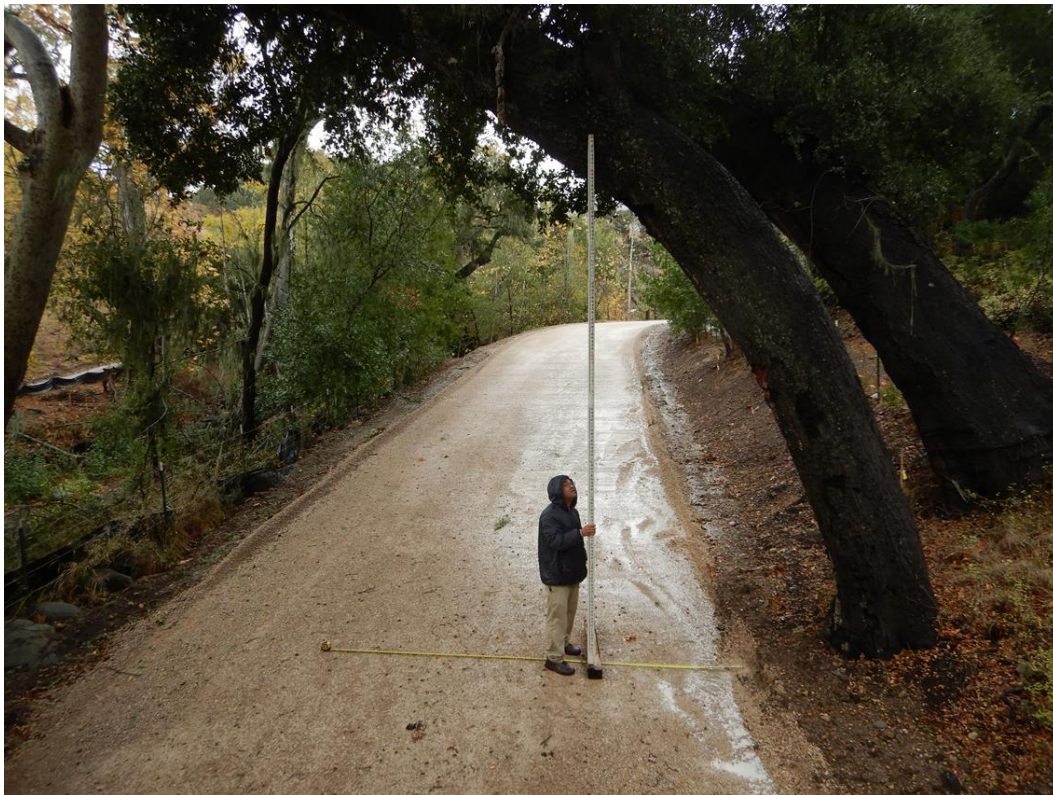
Figure 7: Removal of tree due to road clearance problems.
