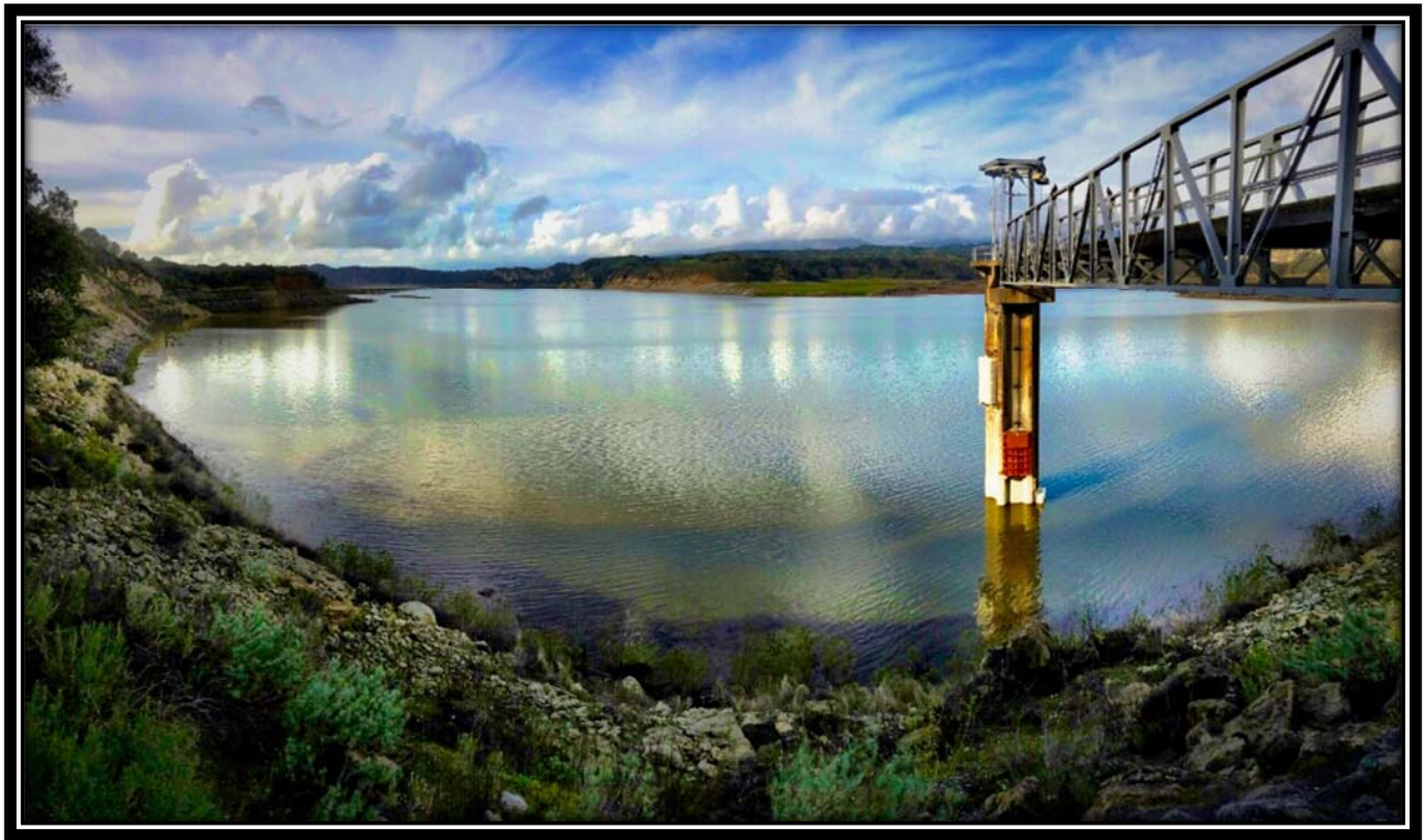
Cachuma Lake – North Portal Intake Tower, February 2017 Photo Credit: D. Flora
