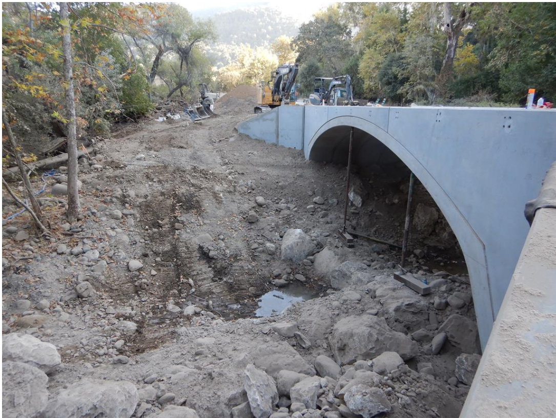
Figure 3: Installed additional RSP.
