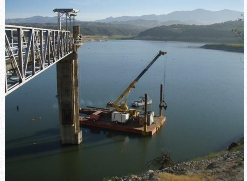
Dredging near Lake Cachuma Intake Tower 2014-2017.
