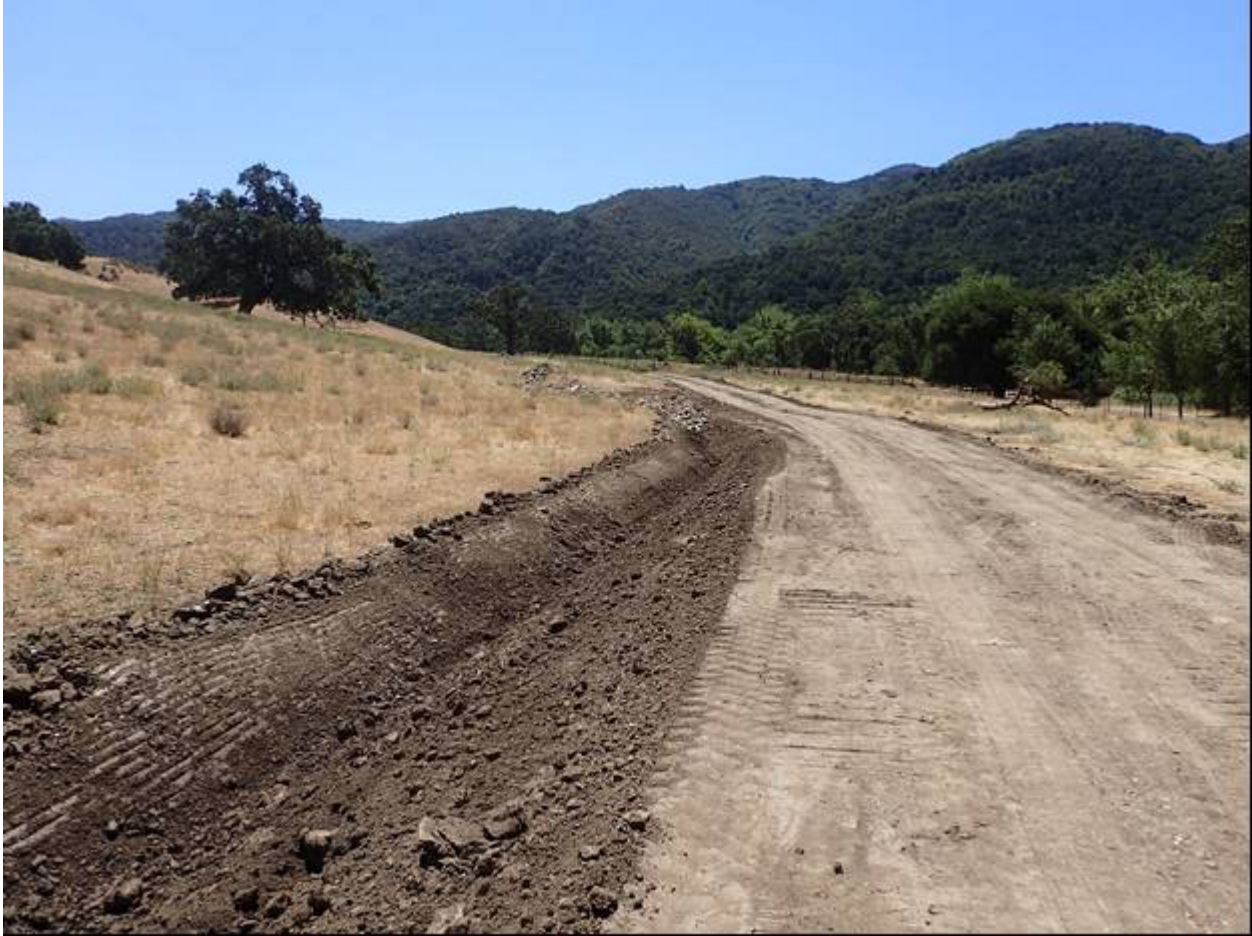
Figure 6: Reconfiguring the Ranch Road drainage.
