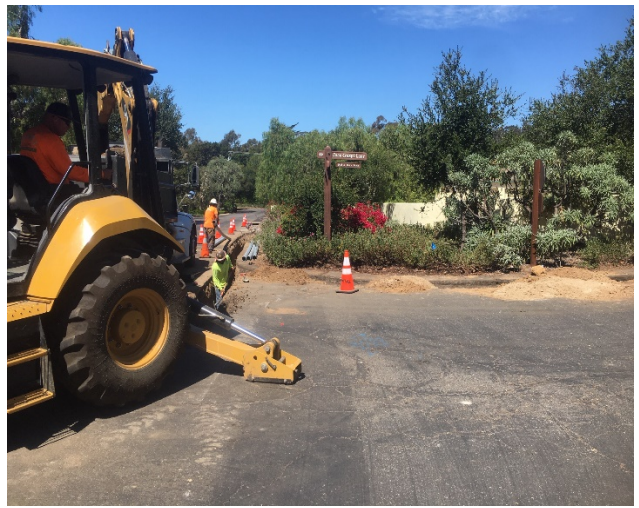
Monitoring Tidwell construction work near the SCC
