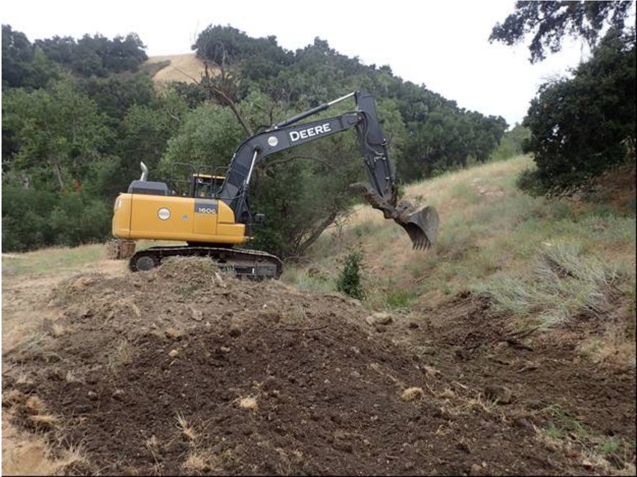
Figure 2: Excavating the settling basin of the no named tributary.
