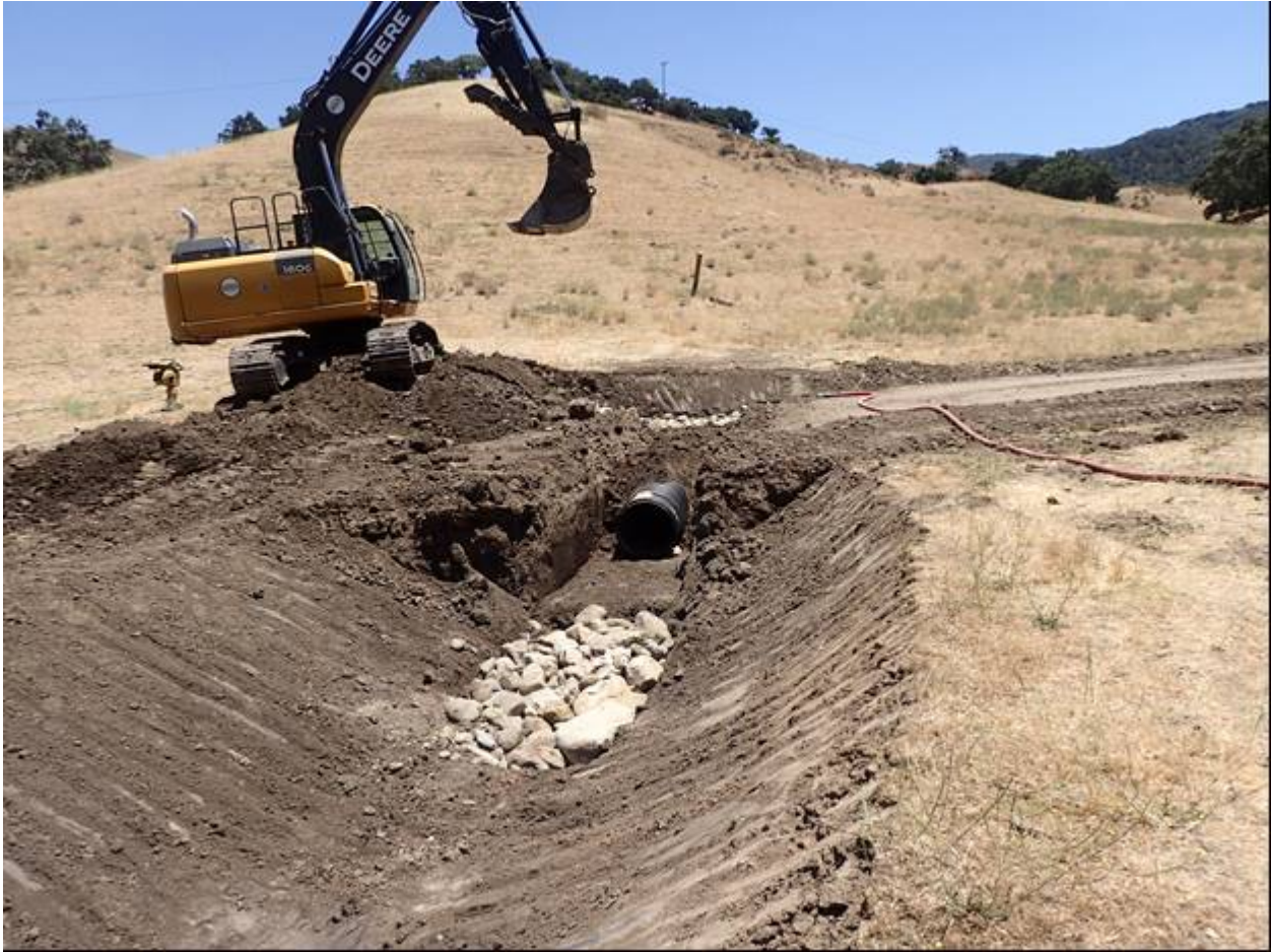
Figure 4: Installing the Ranch Road culvert.
