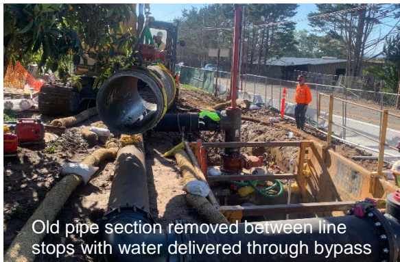
Old pipe section removed - mortar, bar wrapping, and cylinder in excellent condition
