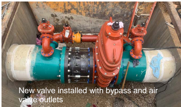
Finished air release valves and valve cans
