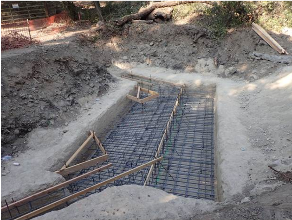
Figure 5: Foundation rebar placement.
