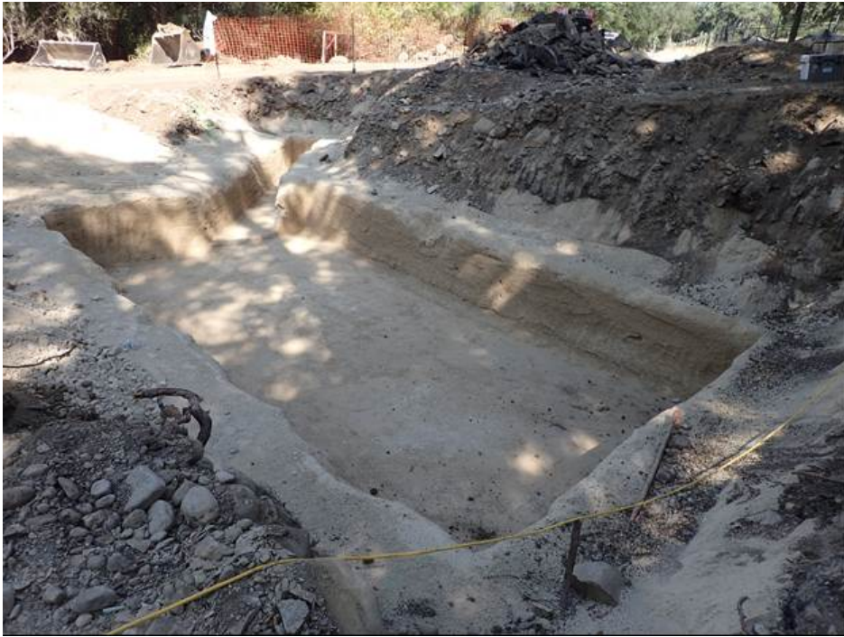
Figure 4: Forming the bridge foundations.
