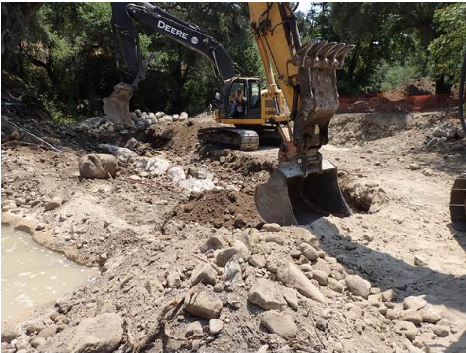
Figure 9: Streambed work, installing the rock slope protection under the bridge.
