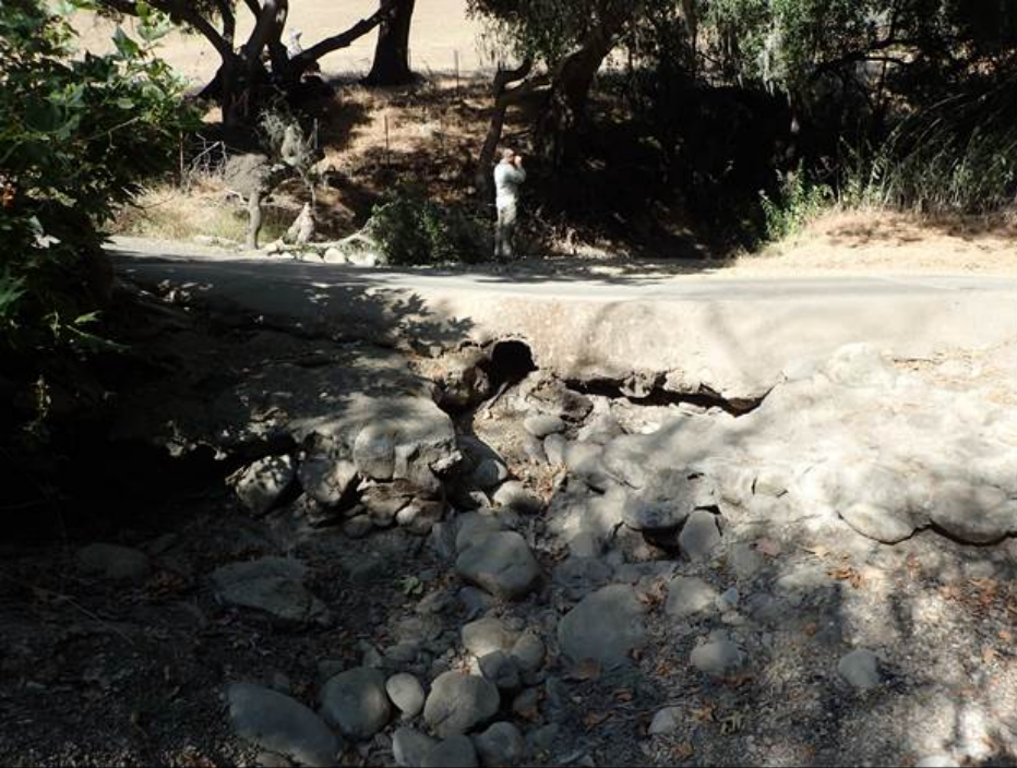
Figure 1: Pre-project condition looking upstream.
