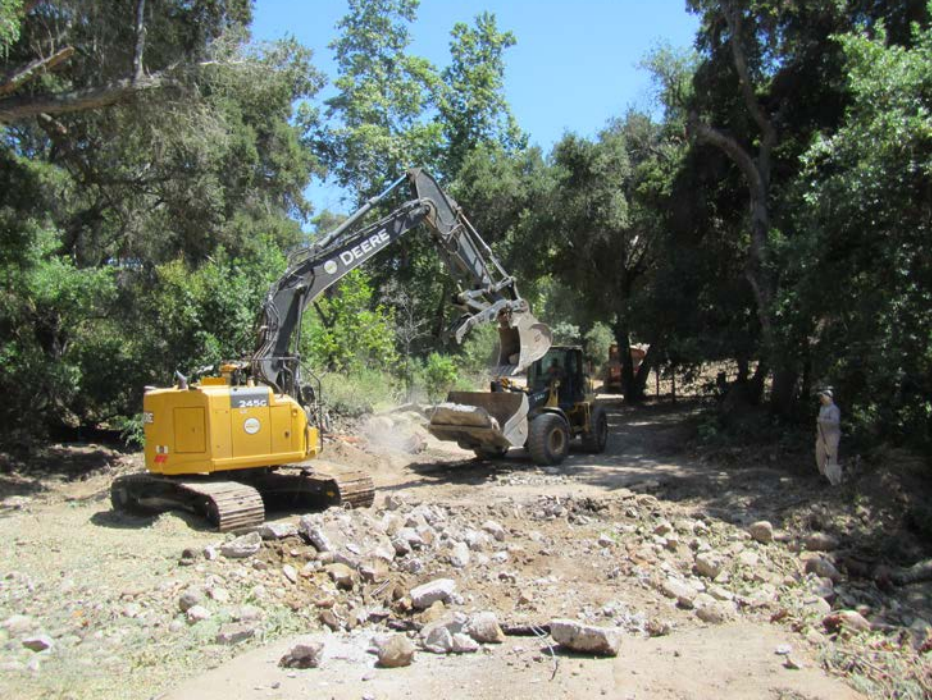
Figure 2: Removal of the concrete low flow crossing along S. Refugio Road.
