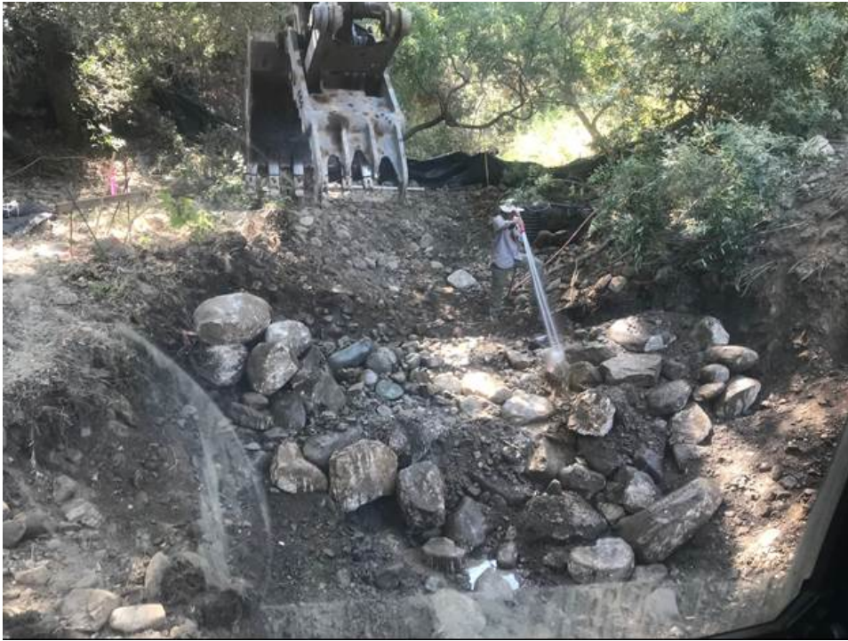
Figure 8: Streambed work, installing the upstream riffle.
