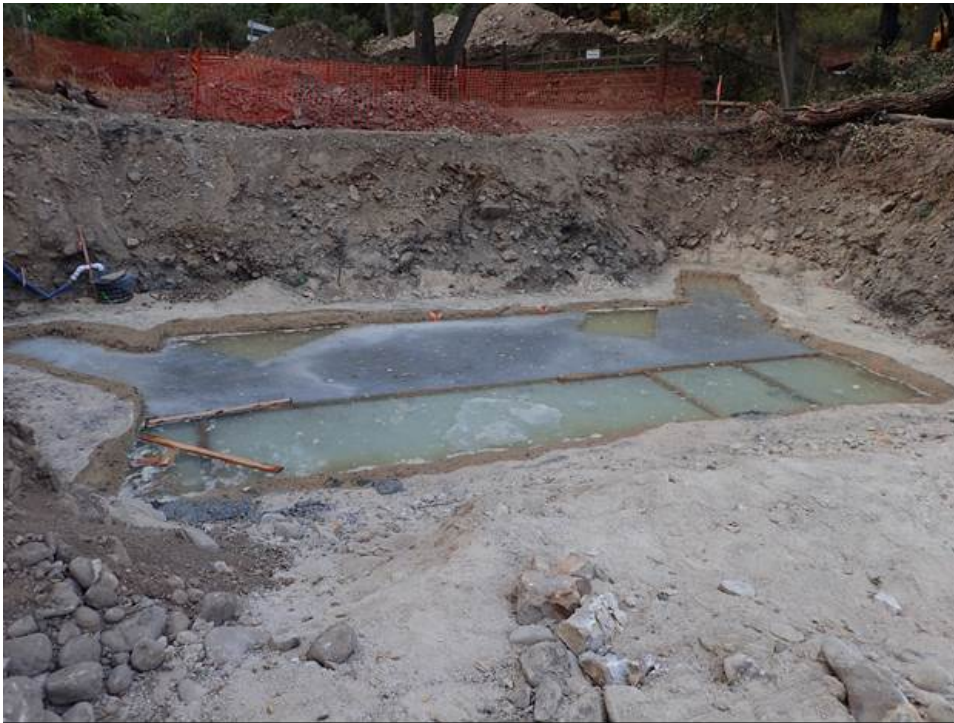
Figure 7: Completed foundation under water for better curing.
