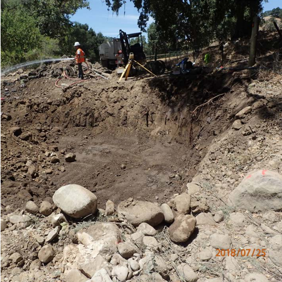
Figure 3: Excavations for the bridge foundations.
