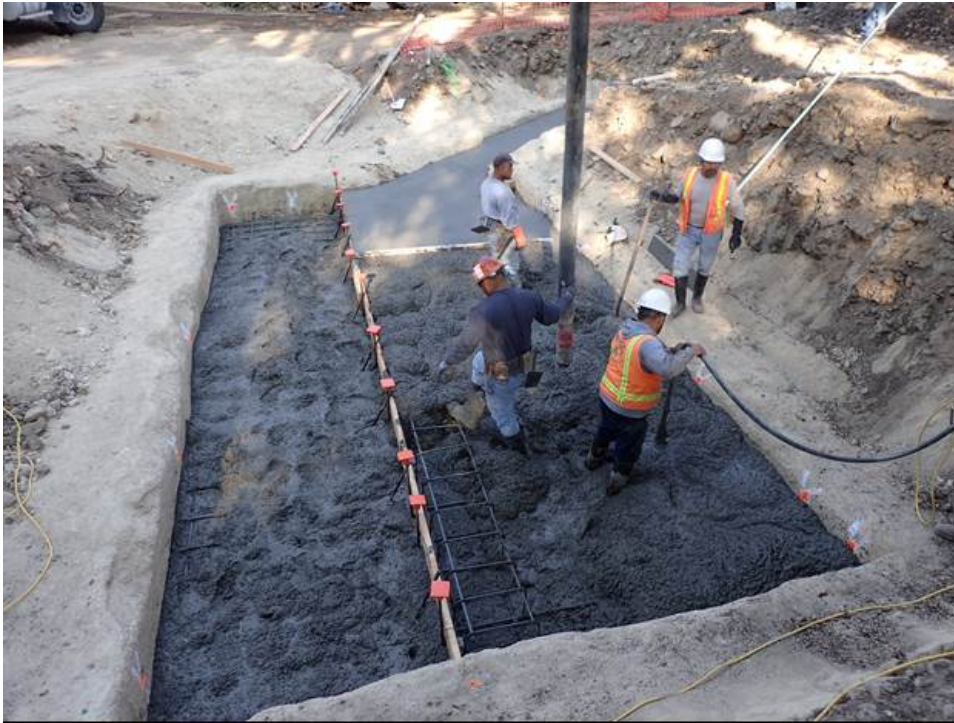
Figure 6: Pouring the foundations.
