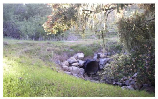
Figure 6-11. El Jaro Creek Demonstration Project: Undersized culvert and ephemeral stream channel
