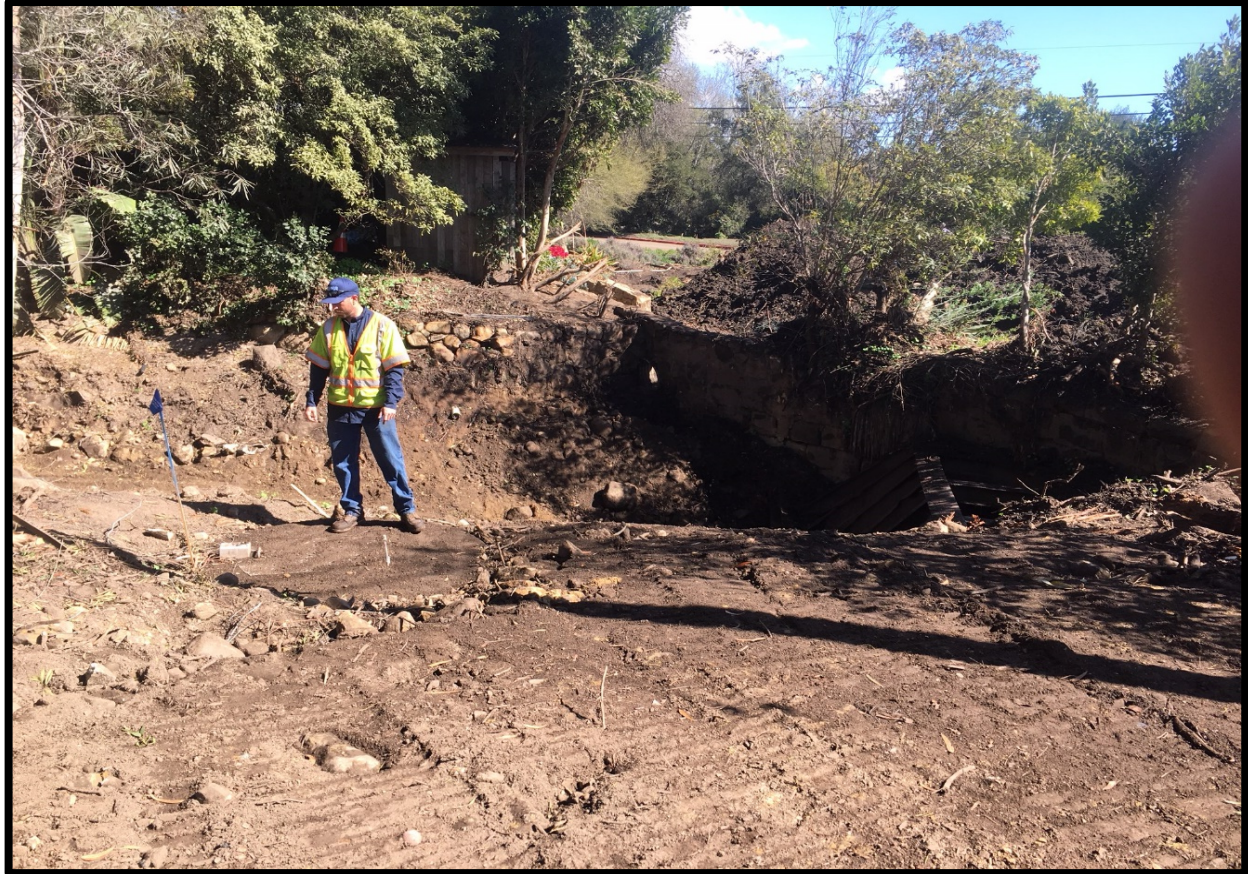
Station #388+10 (Current- Blowoff structure buried)
