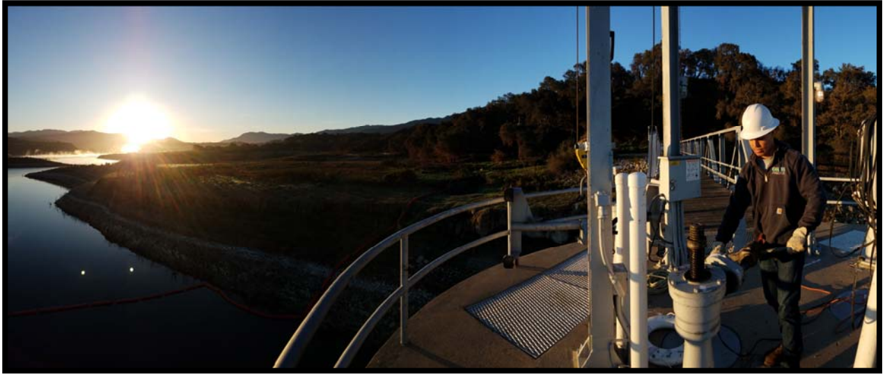
Lake Cachuma Intake Tower slide gate exercising
