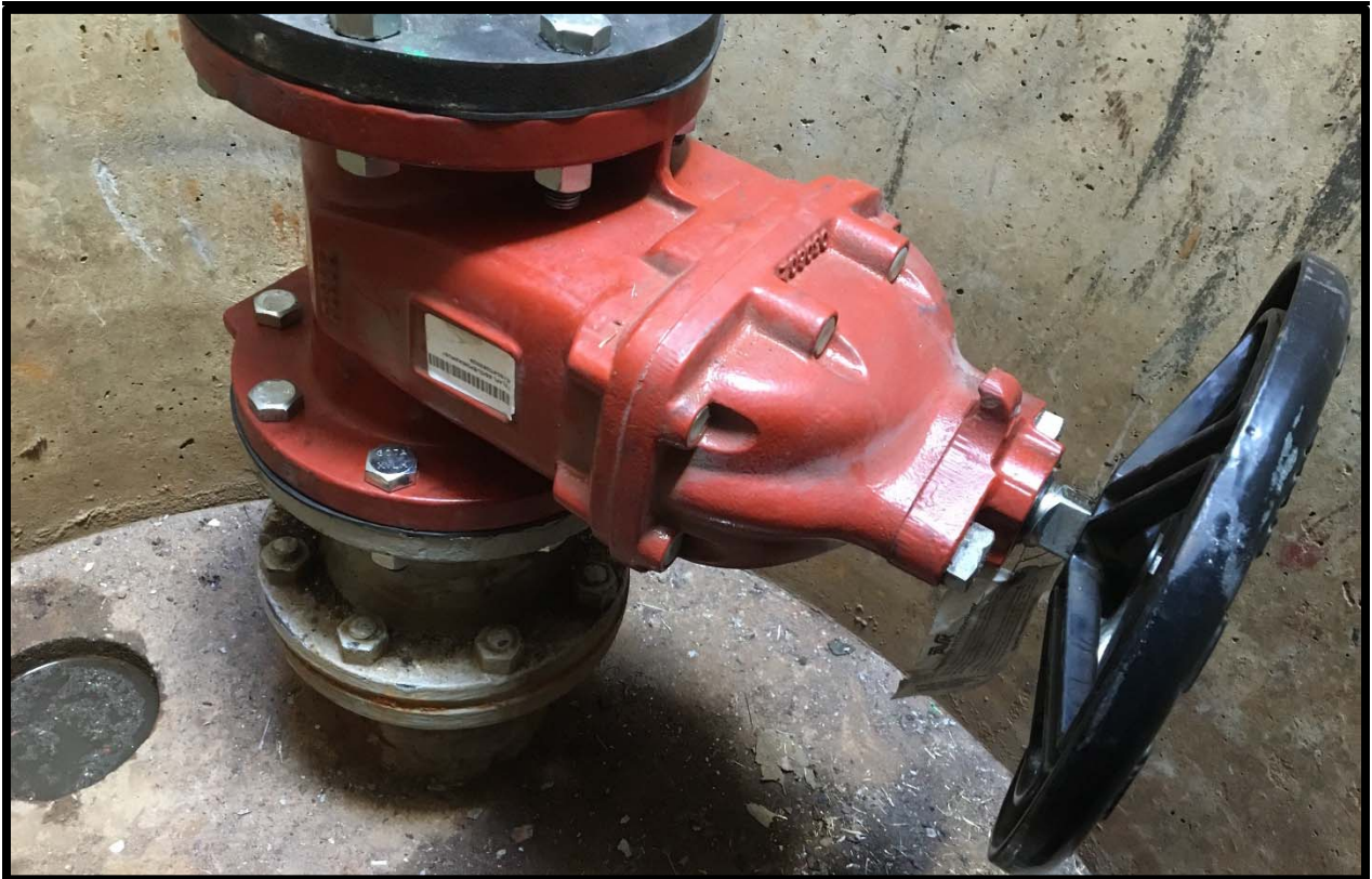
57+97 Valve Replacement and Rehab
