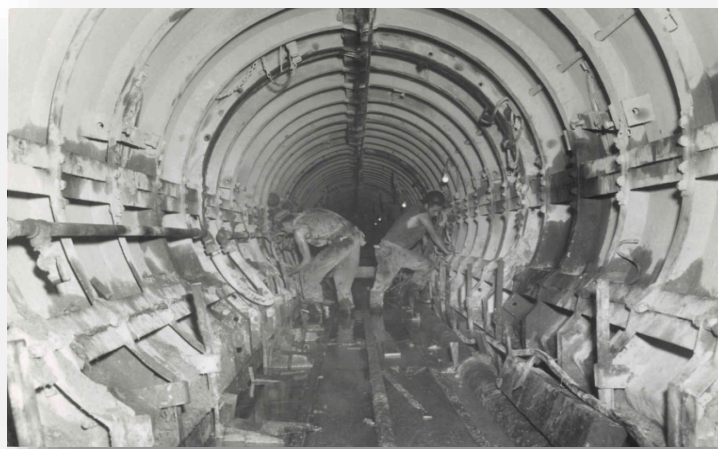
Tecolote Tunnel Construction
