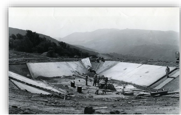
Construction of Bradbury Dam
