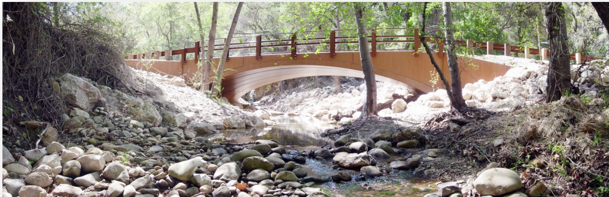
Quiota Creek Fish Passage Project
