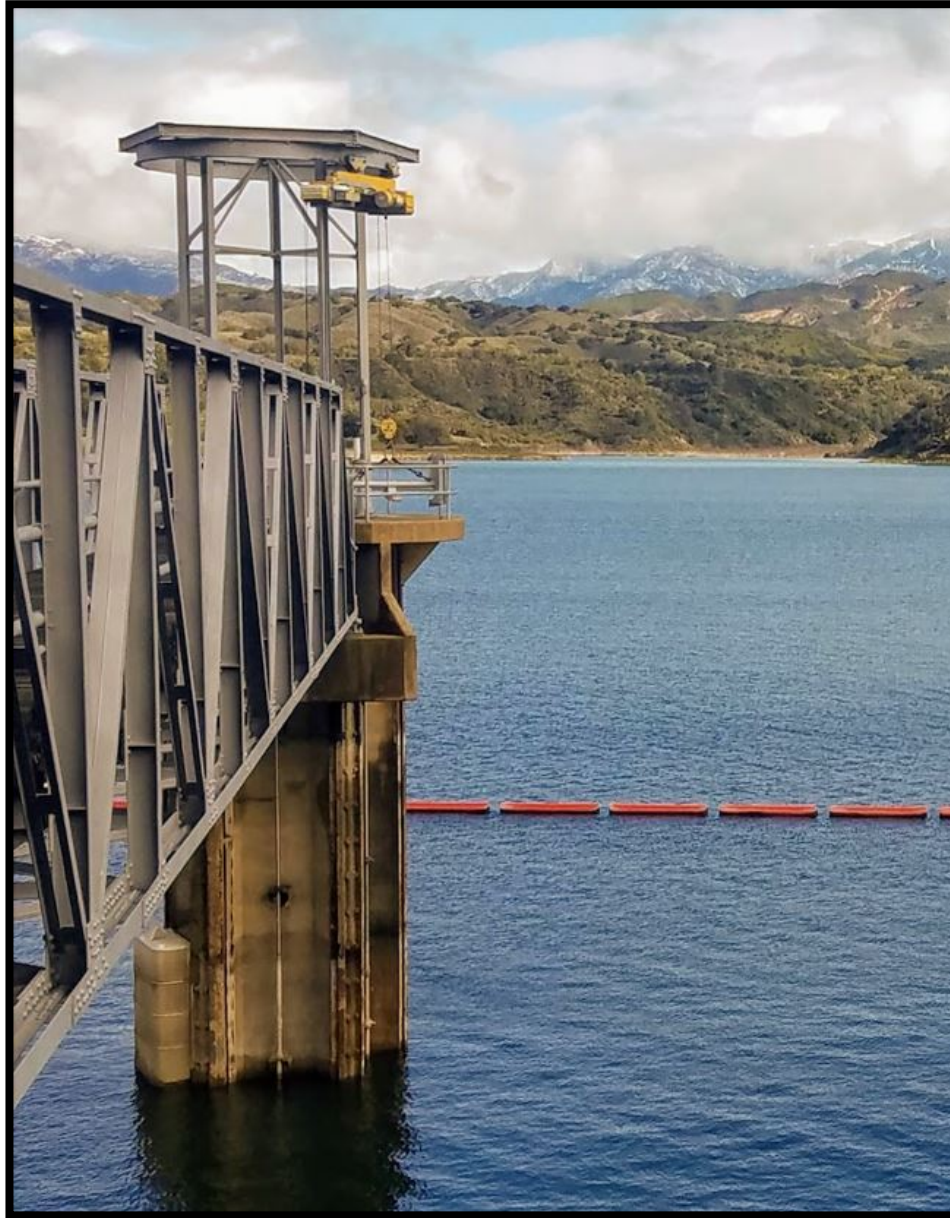
Lake Cachuma, North Portal Intake Tower
