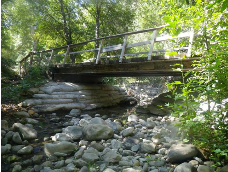
Figure 4: Quiota Creek on Refugio Road showing upstream view of Crossing 8.
