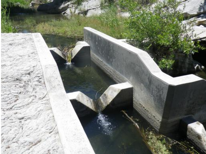
Figure 7: Salsipuedes Creek fish ladder at Jalama Road showing weirs that need to be fixed.
