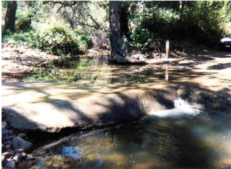
Figure 2: Quiota Creek on Refugio Road showing upstream view of Crossing 4.
