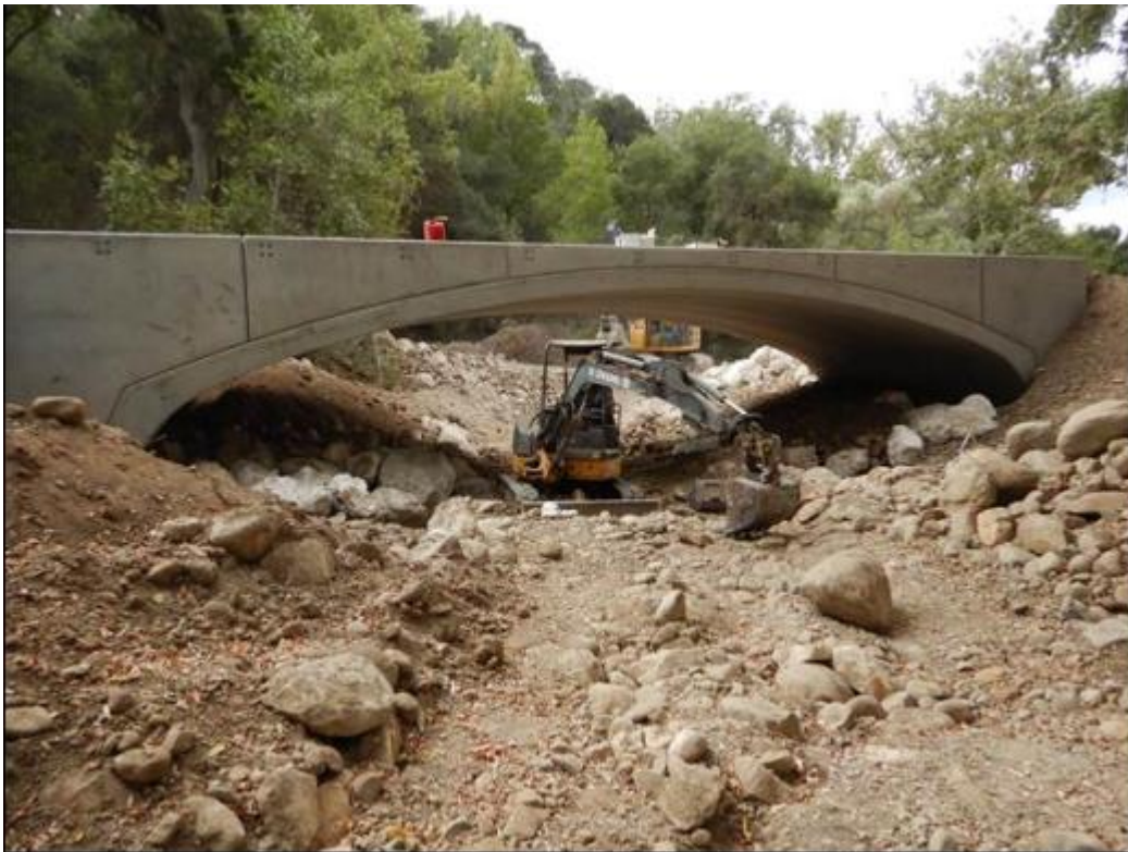
Figure 4: Placing foundation scour protection under the bridge.
