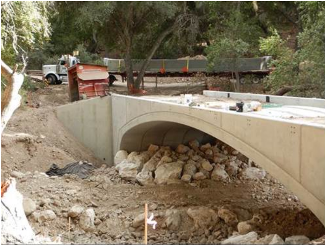
Figure 6: Bridge delivery of the first arch passing around the Quiota Creek Crossing 5 Project site.
