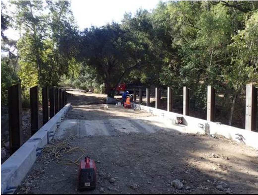
Figure 5: Bridge rail post installation.
