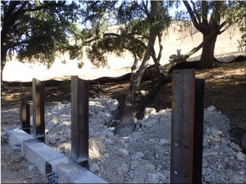
Figure 6: Berm and oak tree rock slope protection.
