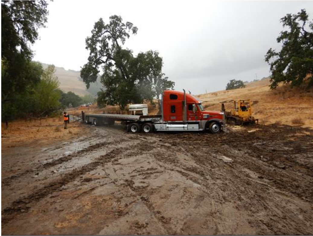
Figure 9: Extracting delivery trucks with a bulldozer.
