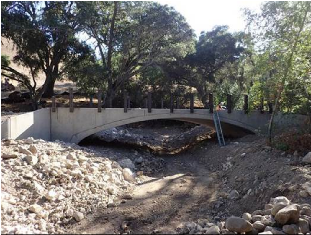
Figure 7: Preparing the bridge for staining and graffiti proofing.
