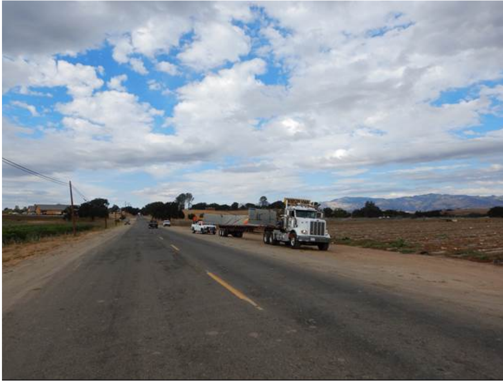
Figure 3: Bridge pieces arrive on 10/2/18.
