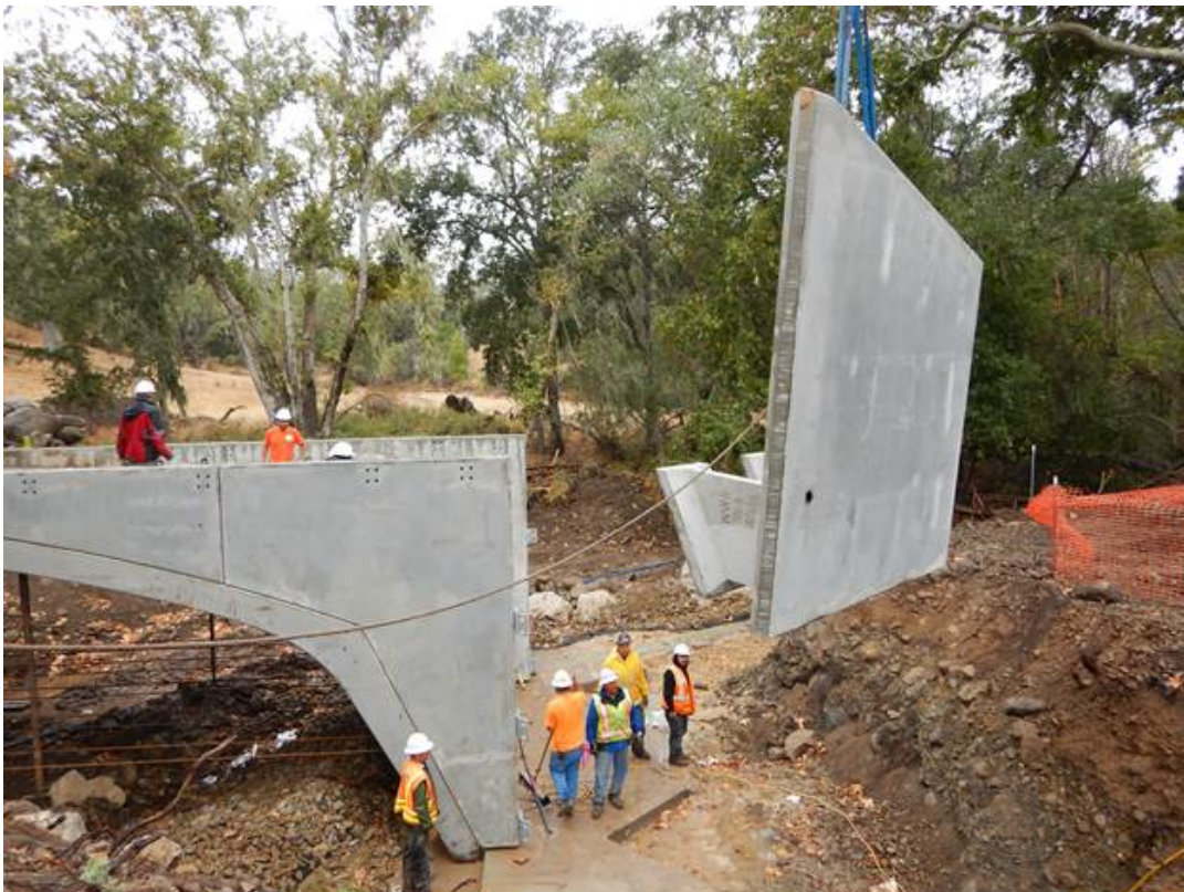
Figure 8: Wing wall installation.
