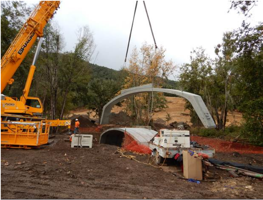
Figure 7: Bridge installation on 10/3/18.
