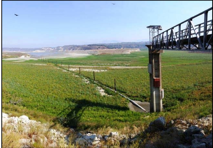
North Portal Intake Tower during drought conditions with pipeline connection to emergency pumping system
