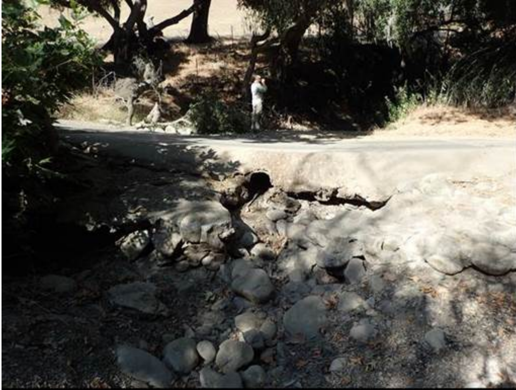
Figure 1: Pre-project condition looking upstream.
