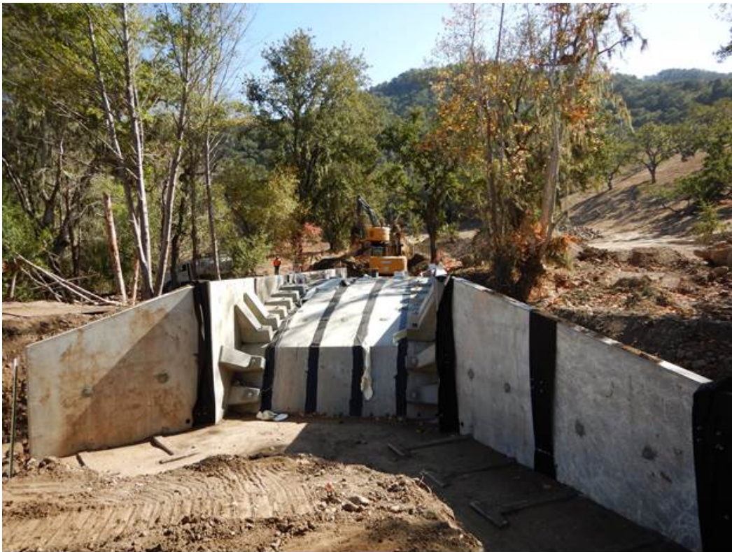
Figure 10: Backfilling the bridge.
