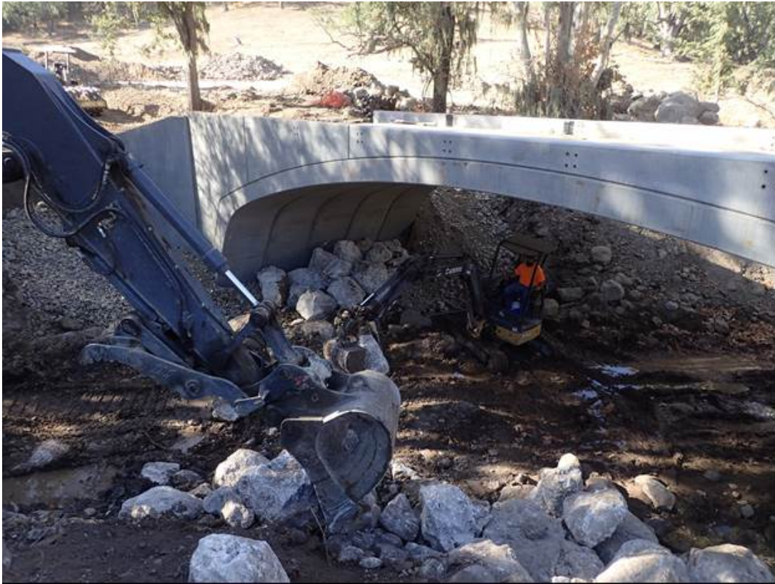
Figure 11: Placing scour protection under the bridge.
