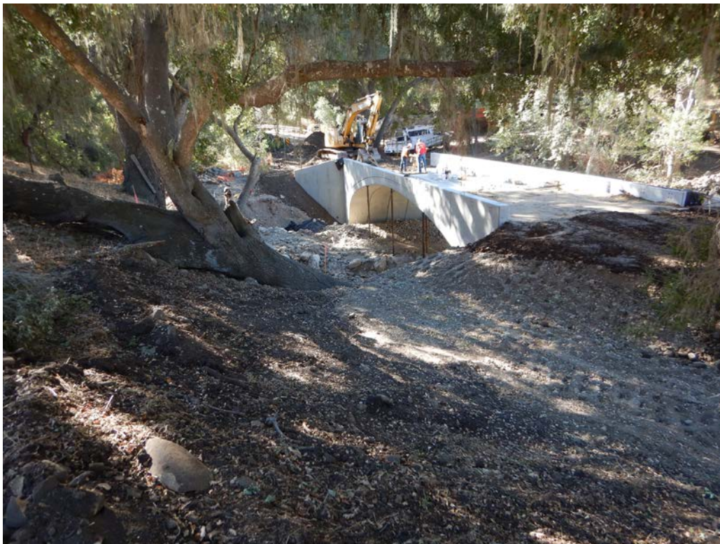
Figure 2: Backfilling the bridge.
