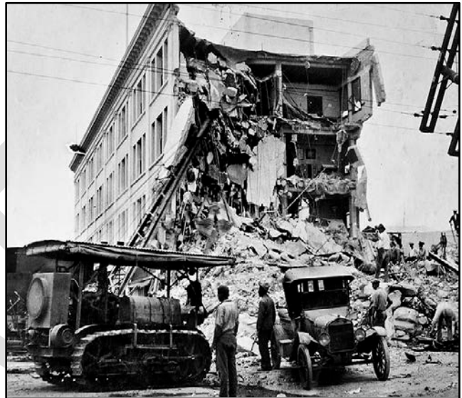
Damage from the 1925 Santa Barbara earthquake
