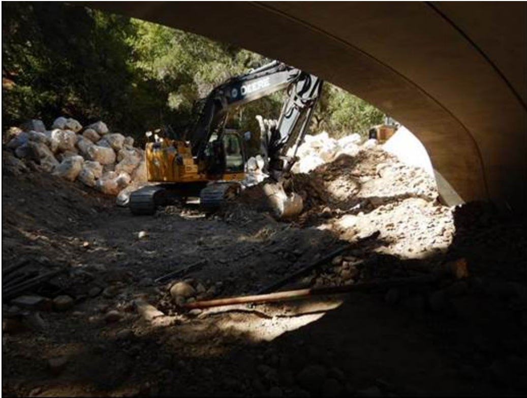
Figure 3: Placing rock slope protection upstream of the bridge.
