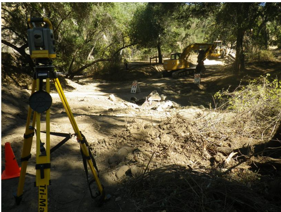
Figure 2: Concrete low flow crossing removal.
