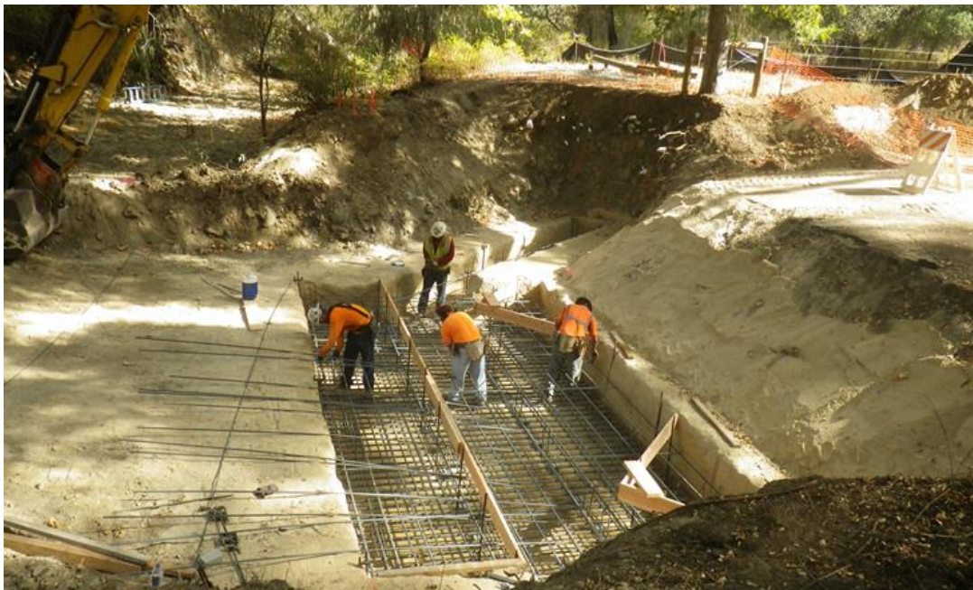
Figure 4: Rebar within the earthen formed foundations.
