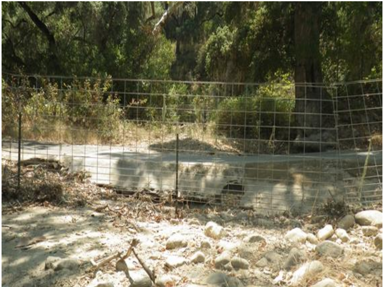
Figure 1: Pre-project condition looking upstream.
