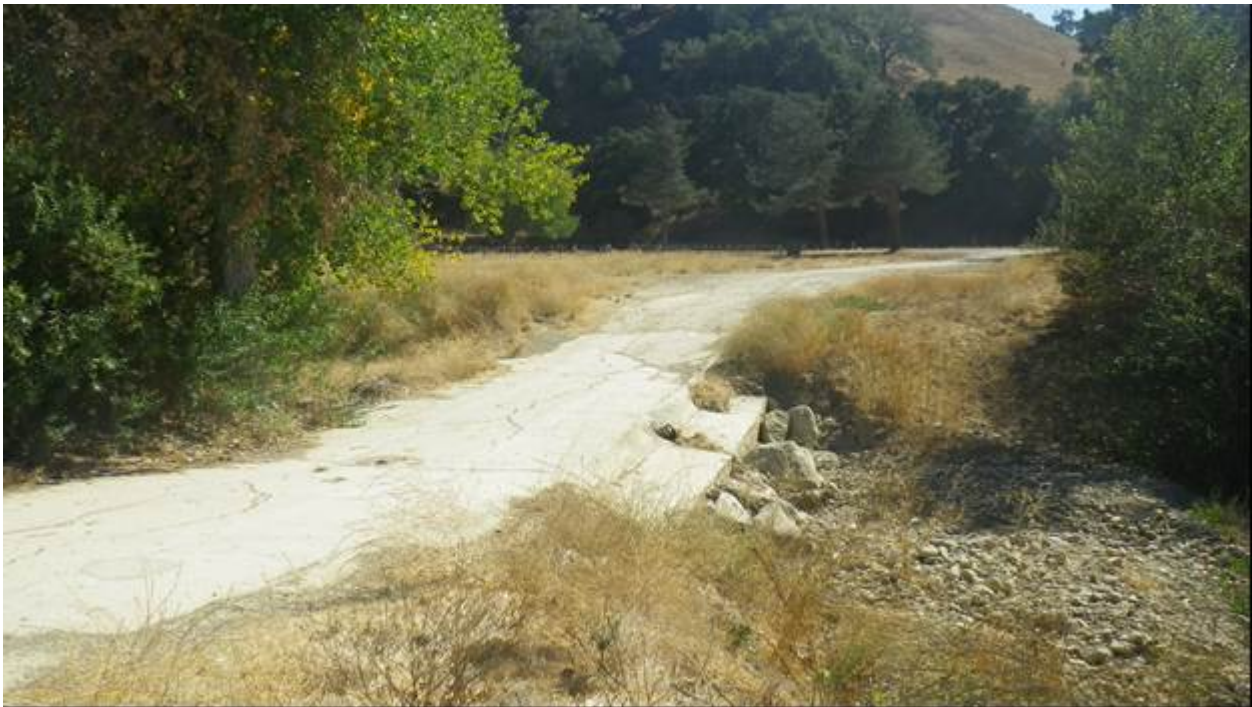
Figure 1: Pre-project condition looking upstream.
