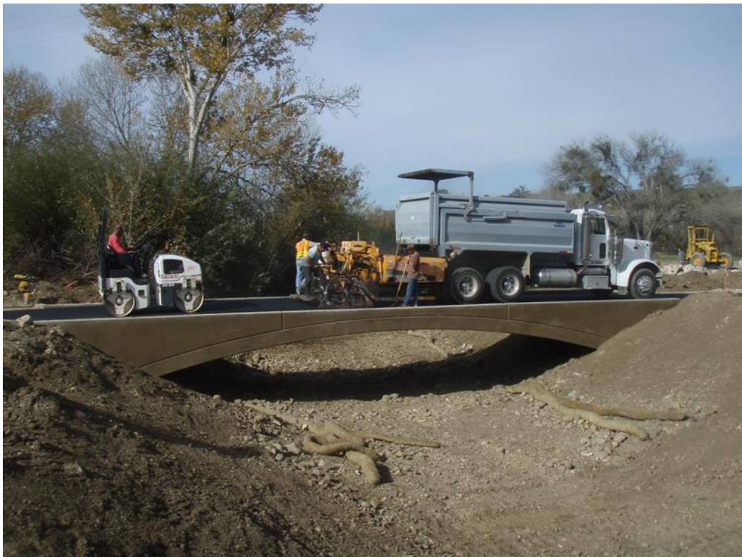
Figure 5: Paving of the road over the bridge.
