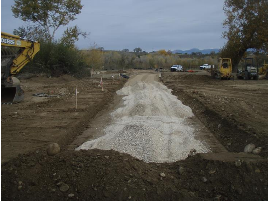
Figure 4: Installing the road base.
