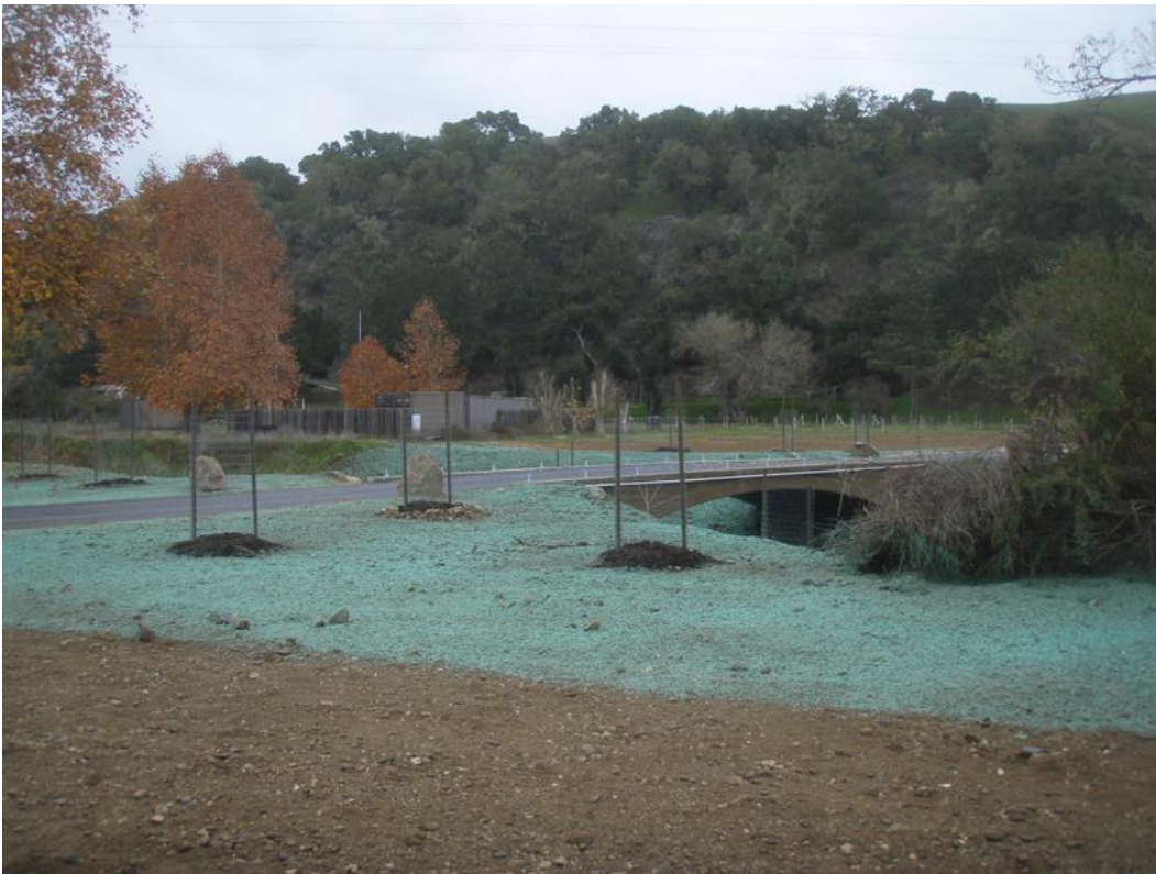
Figure 7: Finished product looking across the bridge.
