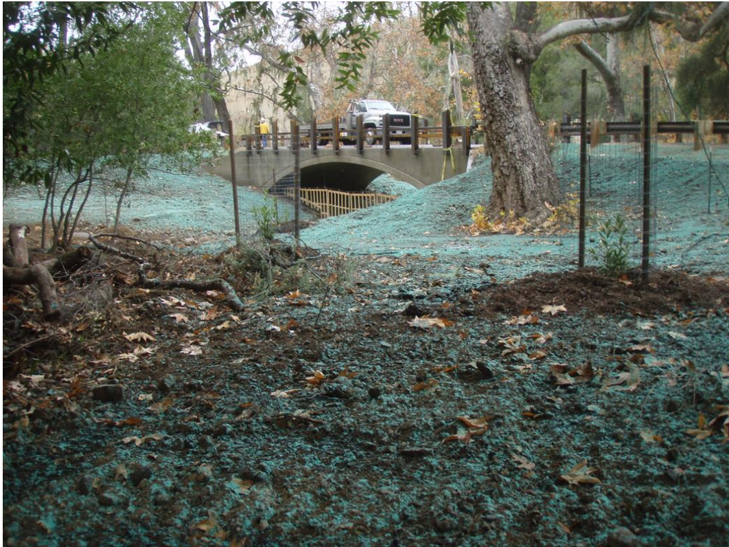
Figure 7: Hydro-mulching/seeding and a near complete project.
