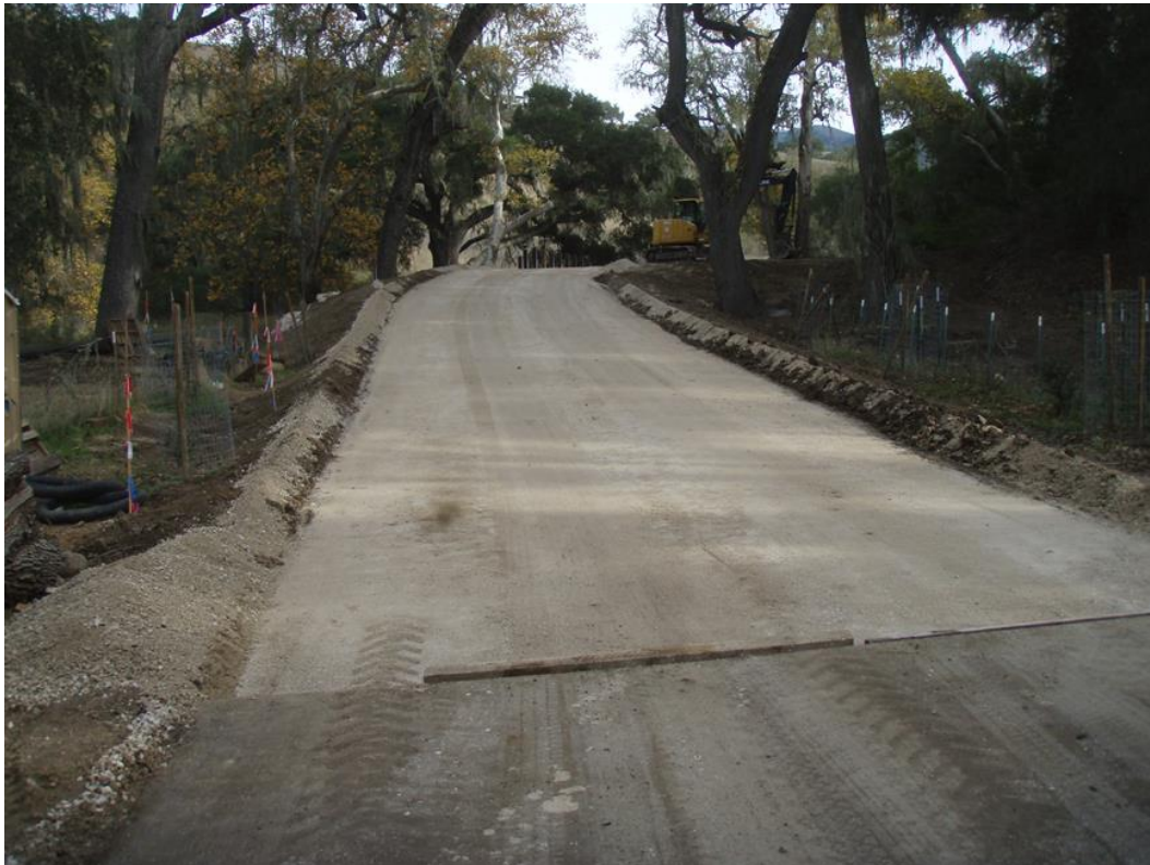
Figure 4: Installation of the road base.
