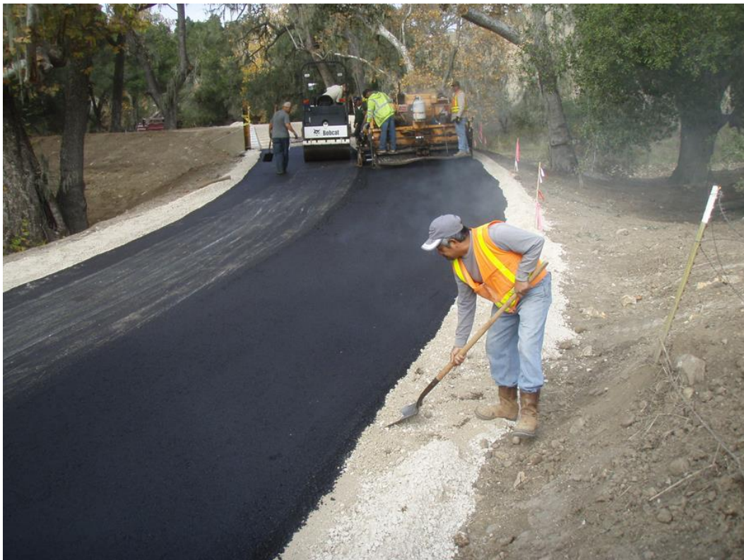
Figure 5: Paving of the road.
