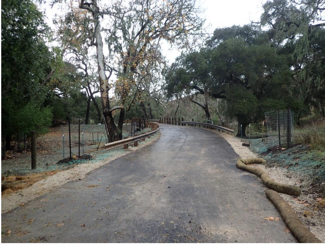
Figure 8: A near complete project.
