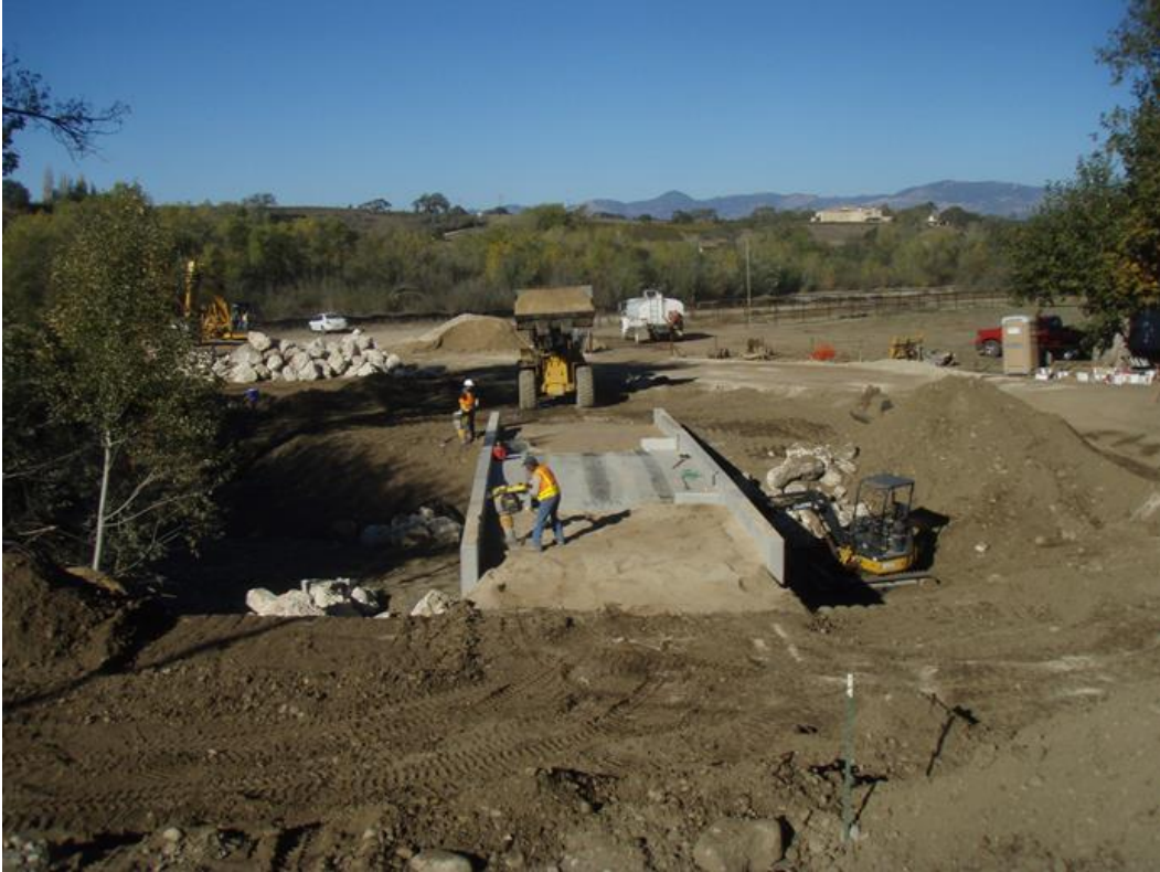
Figure 2: Backfilling of the bridge.
