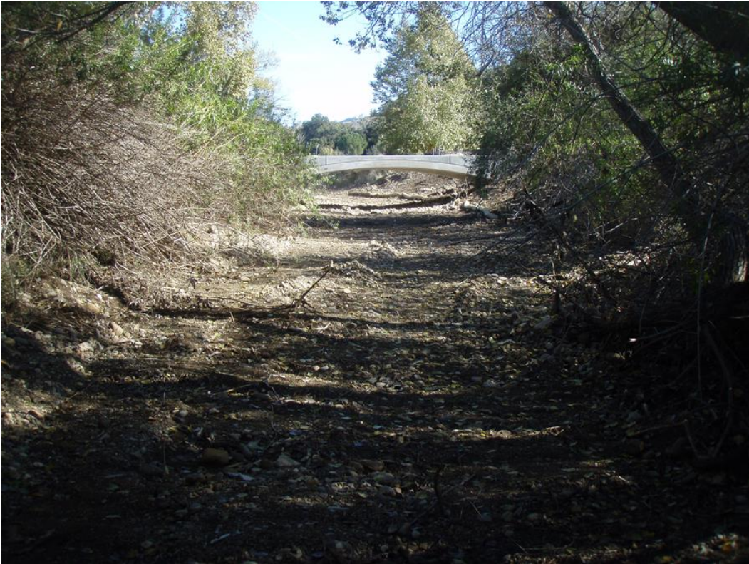
Figure 3: Final stream grading.
