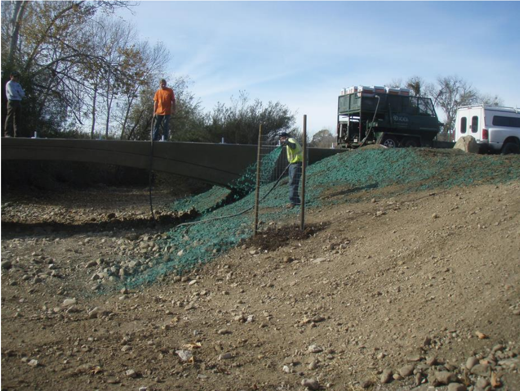
Figure 6: Hydro-mulching and seeding.
