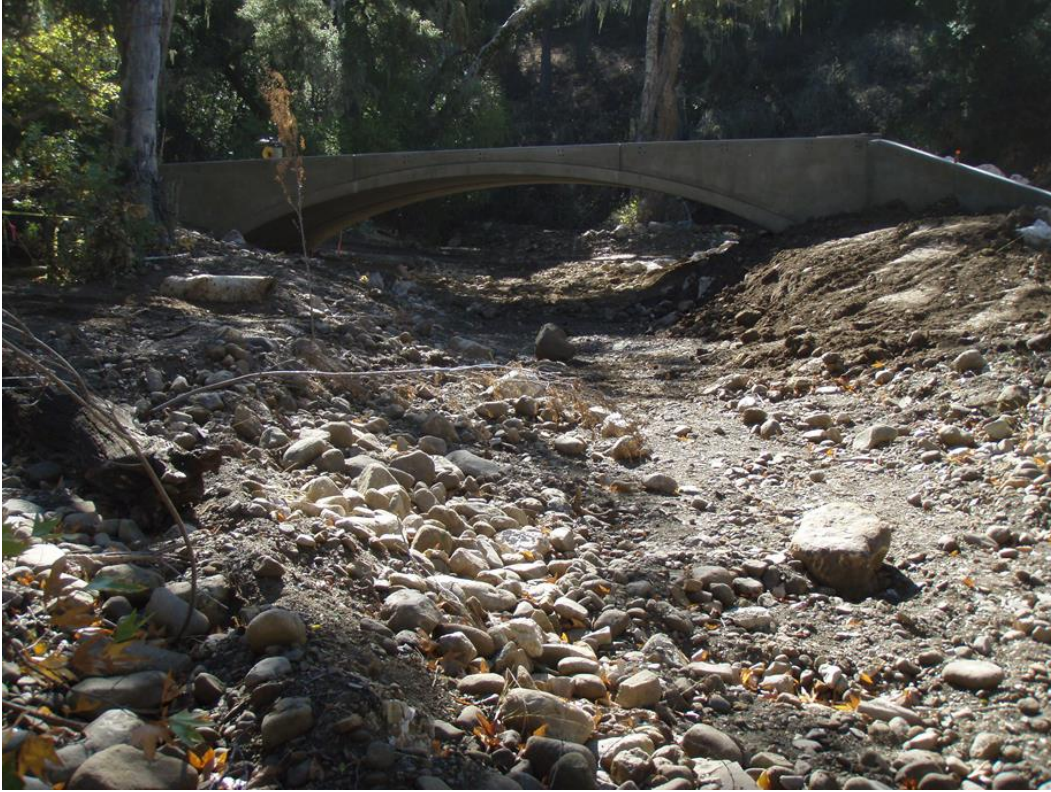
Figure 2: Final stream grading.
