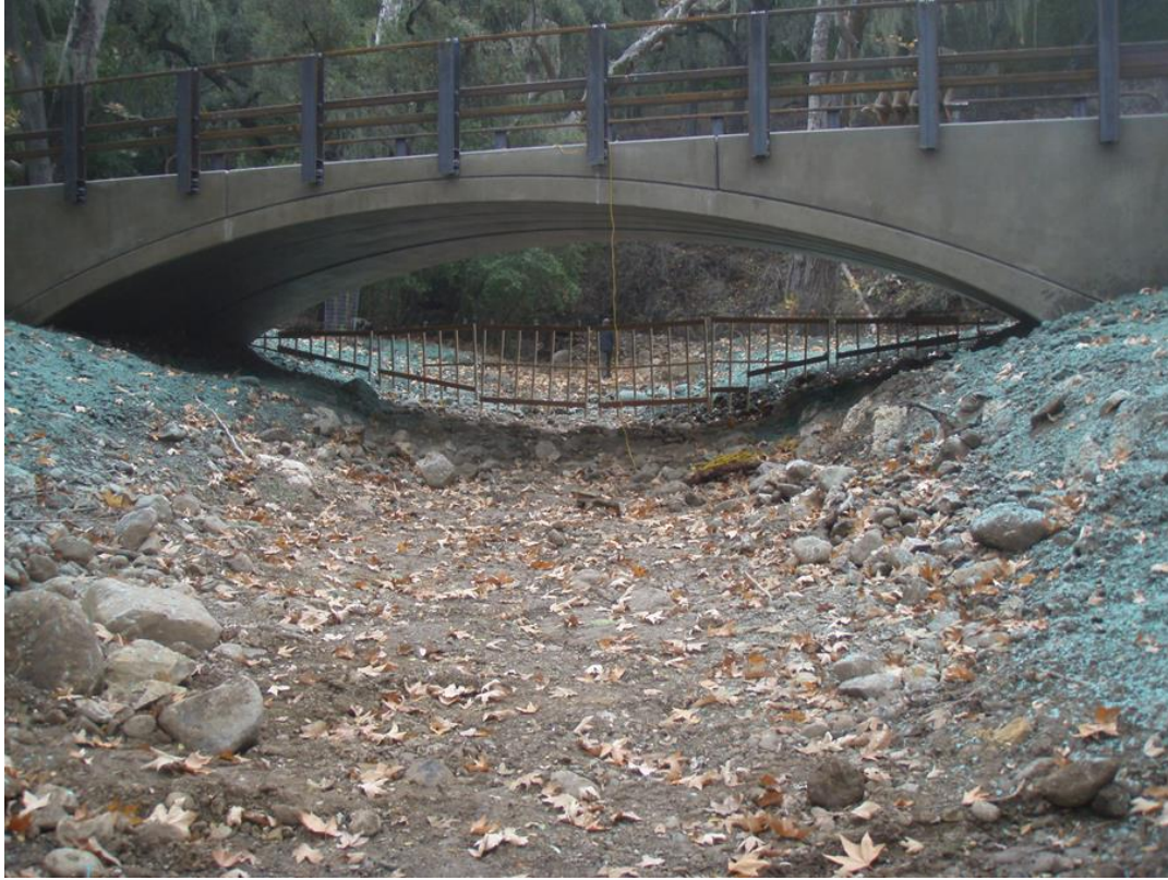
Figure 6: Installation of the Bridge rail and guardrail.
