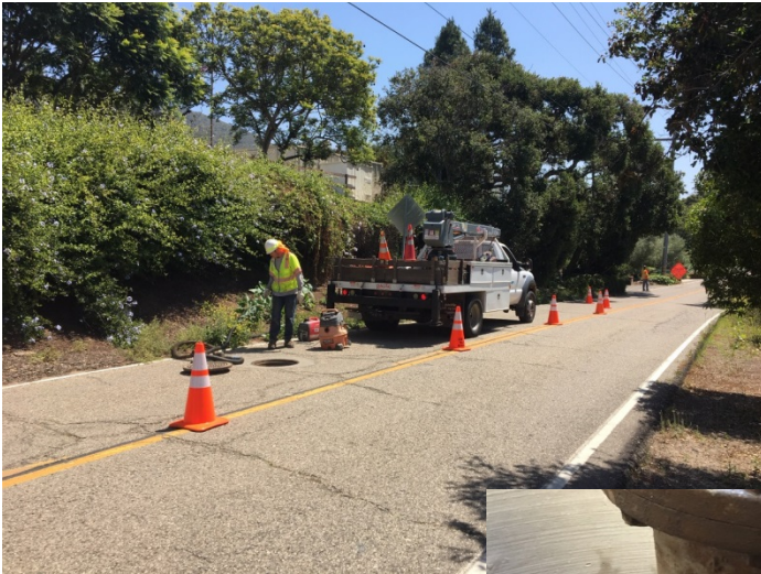
Traffic control required in street
