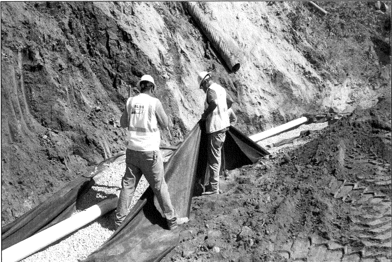
Installing subdrain in fill slope
