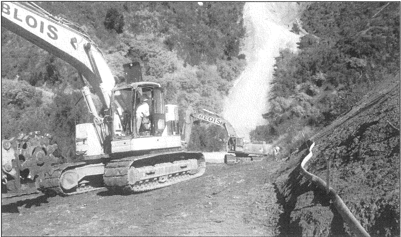
Finish grading and compacting slope up to Glen Annie Turnout
