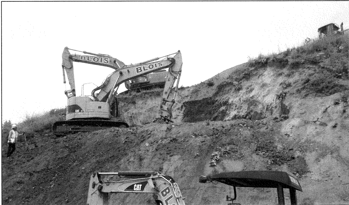
Completing construction of structural fill slope
