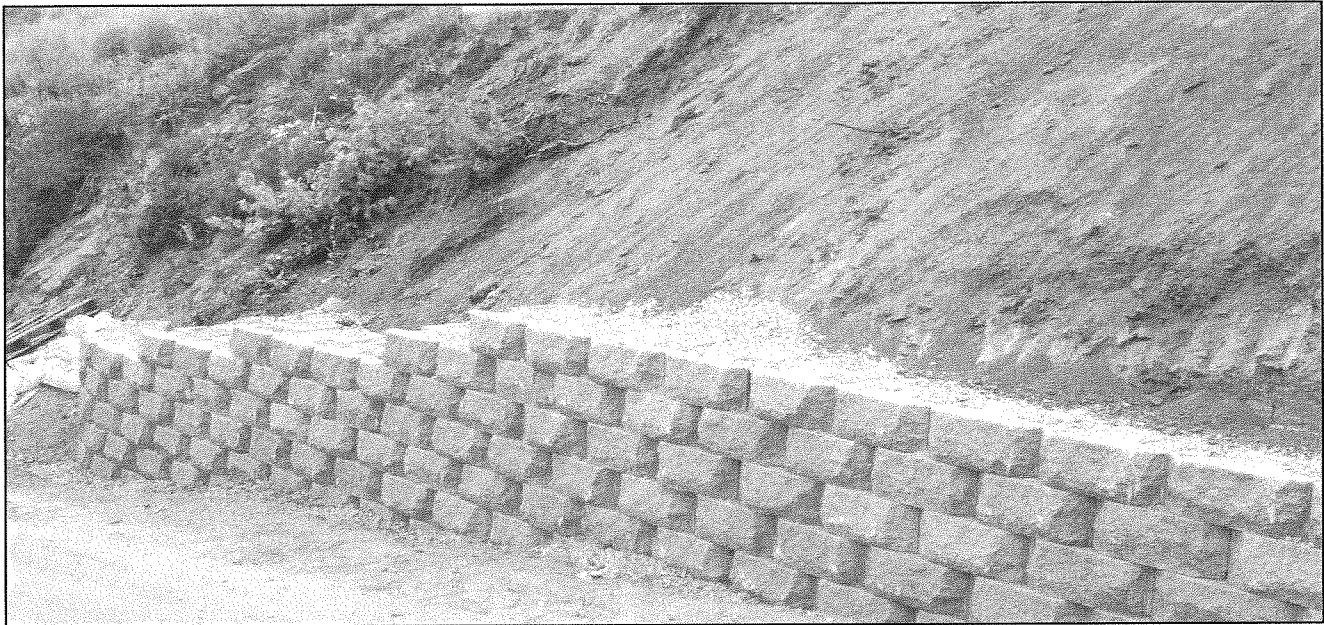
Gravity Block Retaining Wall
