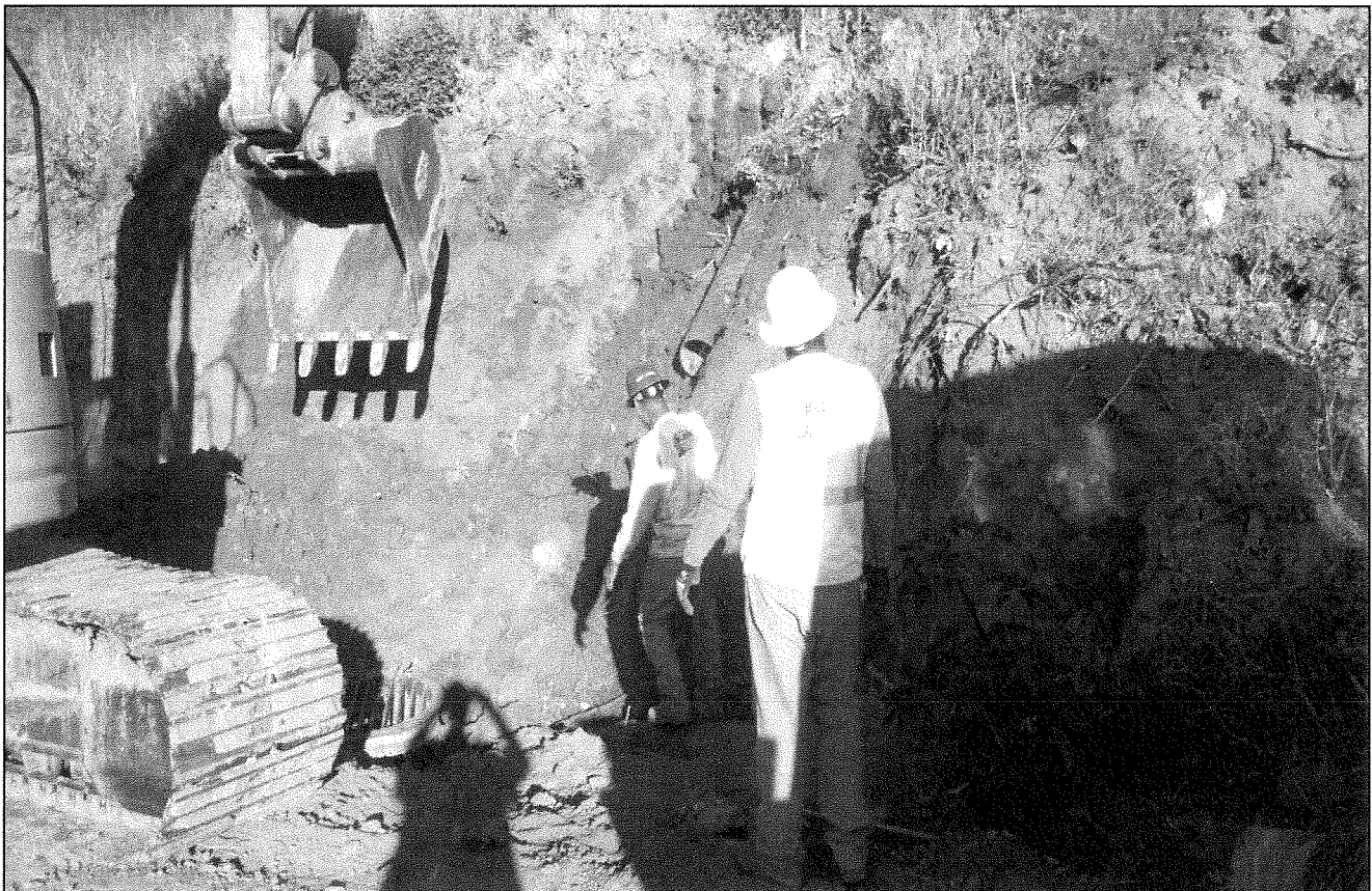
Excavating key for fill slope above Glen Annie Turnout Access Road
