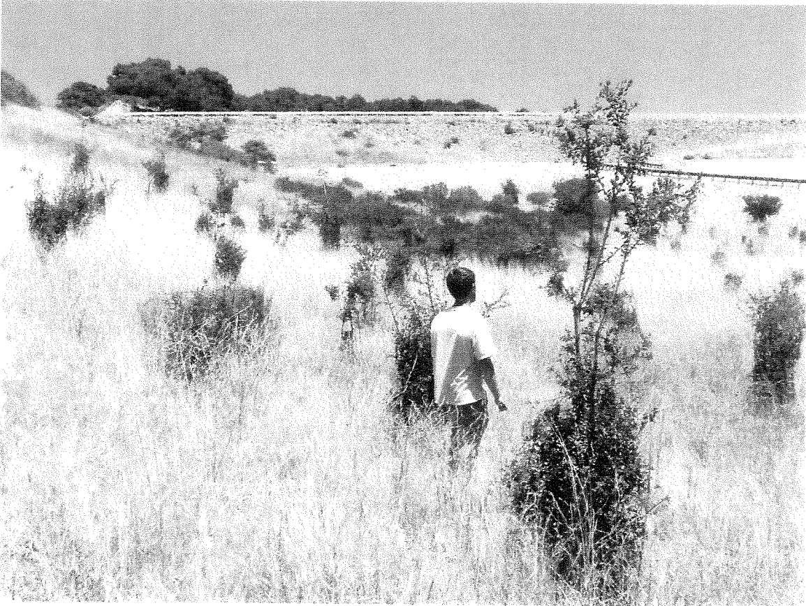
2012 at Bradbury Dam, South facing slope
