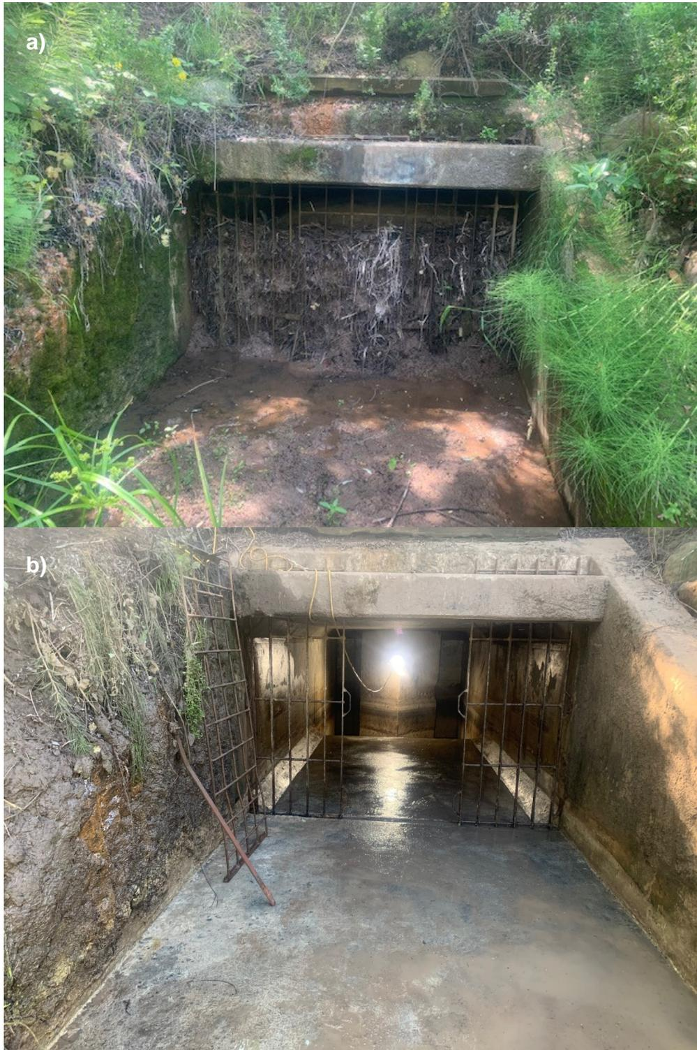
**Figure 1.** Lauro Reservoir Spillway Stilling Well (a) debris deposited during 2023 winter storms; (b) stilling well post debris removal.
