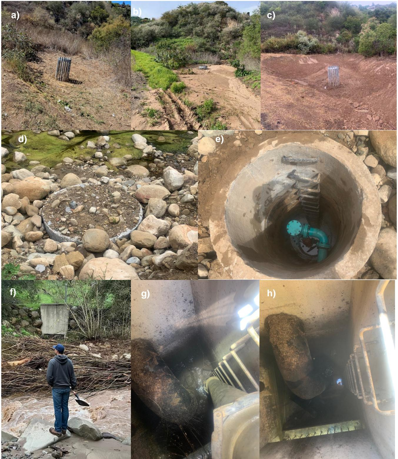
**Figure 2.** County-Wide Debris Removal related to 2023 Winter Storms Project Costs – San Roque Debris Basin (a) pre-storm), (b) post-storm, (c) post debris removal; Toro Canyon Blowoff (d) post-storm, (e) post debris removal; Carpintera Toe Drain (f) post-storm, (g) during debris removal, (h) post debris removal.
