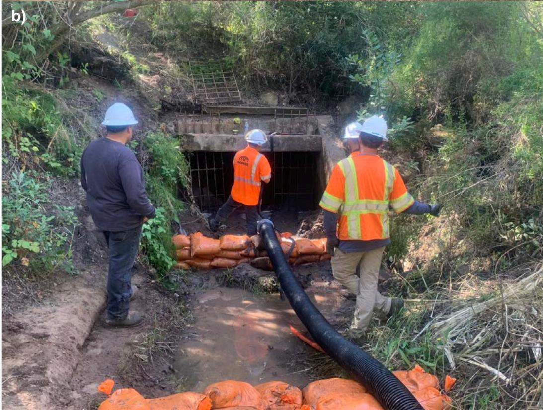
**Figure 2.** Lauro Reservoir Spillway Stilling Well (a) combination hydrojetting vacuum truck utilized to remove debris; (b) 300 feet of 6-in corrugated HDPE pipe utilized to transport vacuumed sediment and water and sandbag dams utilized to contain the sediment.
