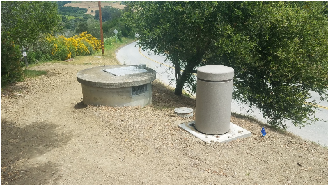
Lower Reach Structure Maintenance – Clearing vegetation from structures
