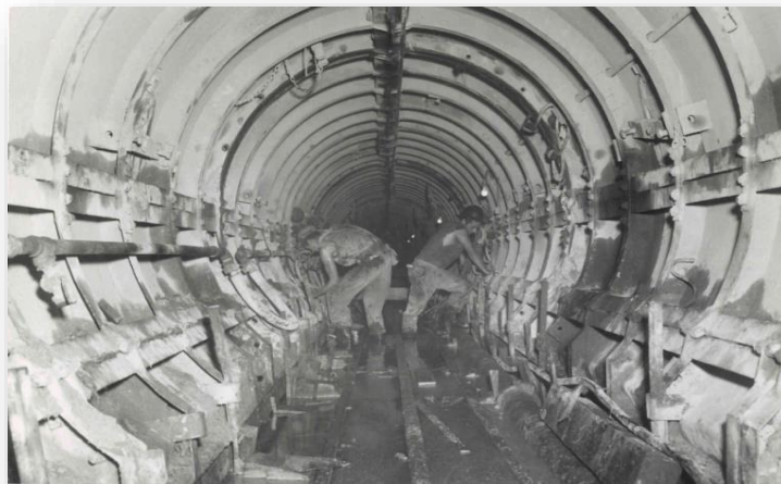
Tecolote Tunnel Construction
