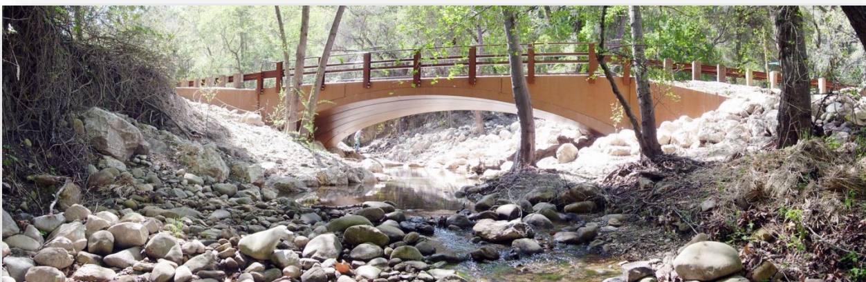
Quiota Creek Fish Passage Project
