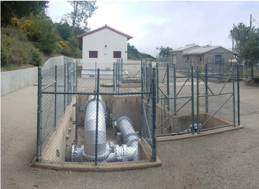
Ortega Valve Pit #1 – Pit cleaned, valves painted and actuators greased
