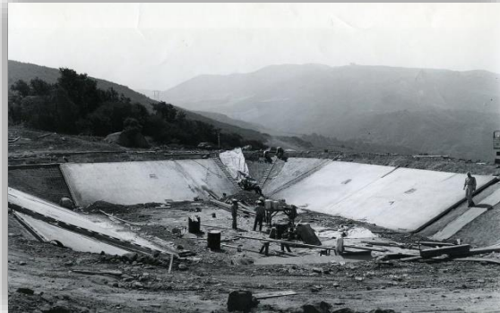
Construction of Bradbury Dam
