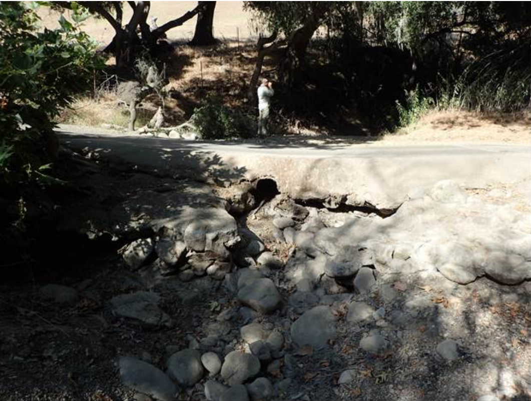
Figure 1: Pre-project condition looking upstream.
