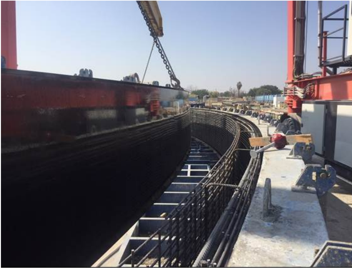
Figure 4: Bridge fabrication (arch) at Bethlehem, Wasco, CA.
