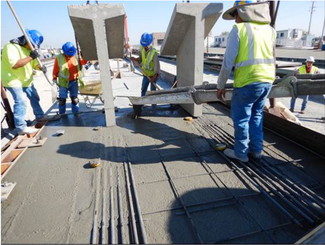
Figure 6: Bridge fabrication (wing wall) at Bethlehem, Wasco, CA.
