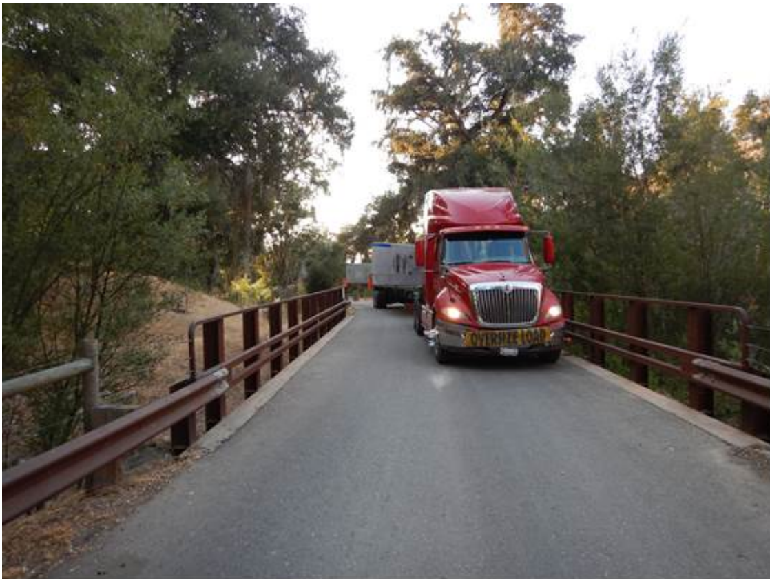
Figure 3: Bridge delivery and navigating S. Refugio Road over the Quiota Creek Crossing 2 Bridge.
