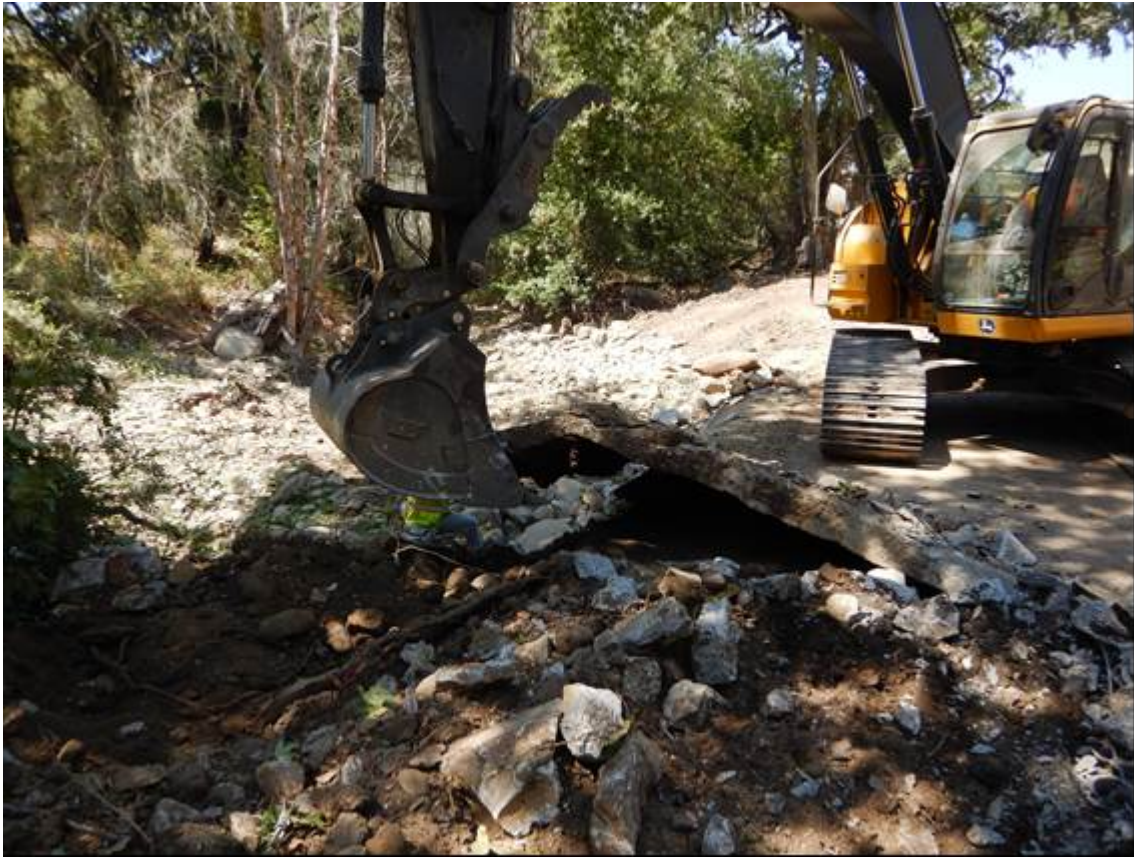
Figure 8: Removing the crossing and conducting biological surveys under the crossing.
