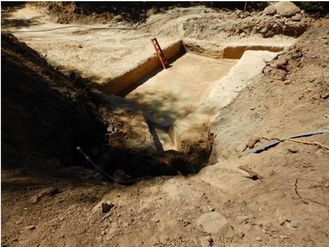
Figure 9: Foundation preparation.
