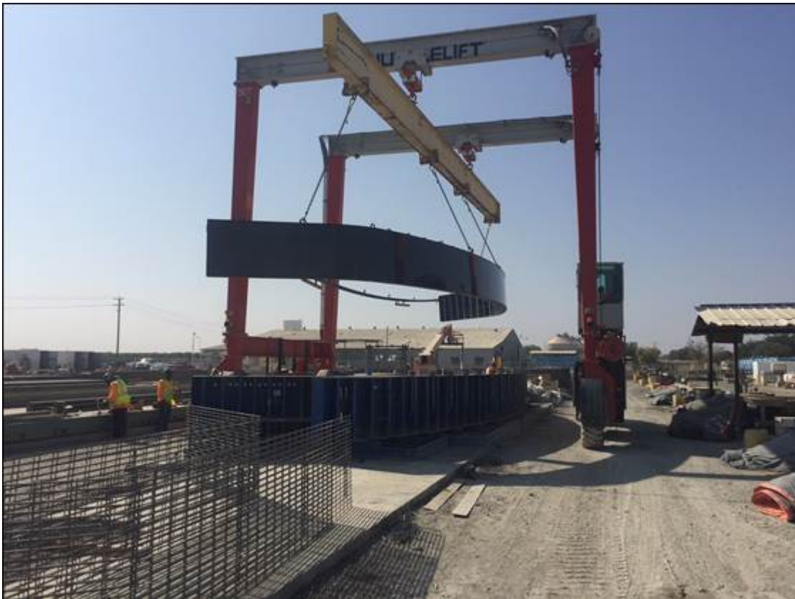
Figure 3: Bridge fabrication (arch) at Bethlehem, Wasco, CA.
