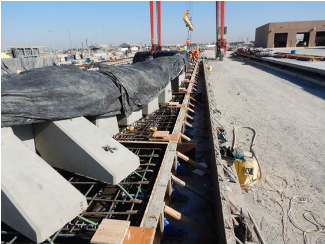
Figure 5: Bridge fabrication (headwalls) at Bethlehem, Wasco, CA.
