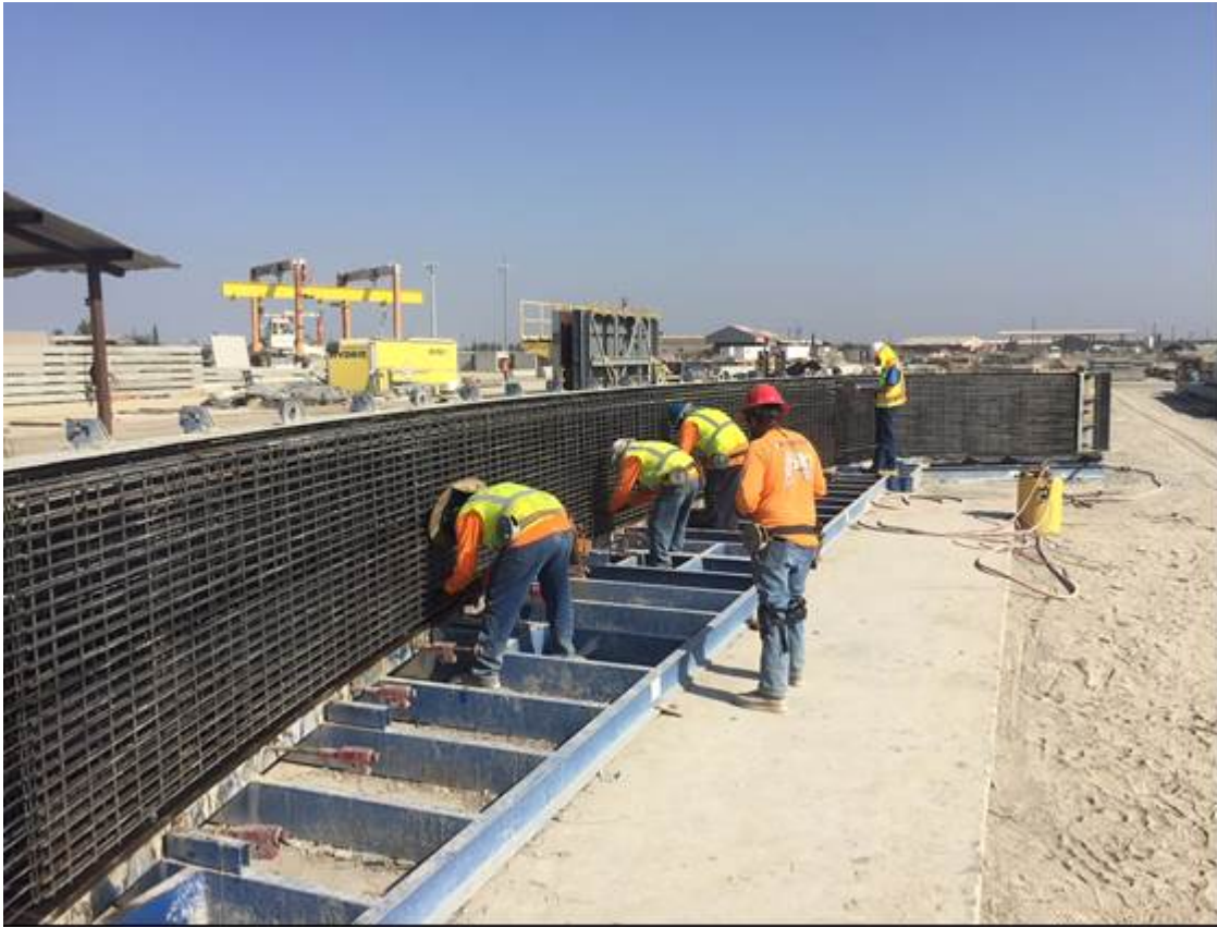
Figure 2: Bridge fabrication (arch) at Bethlehem, Wasco, CA.
