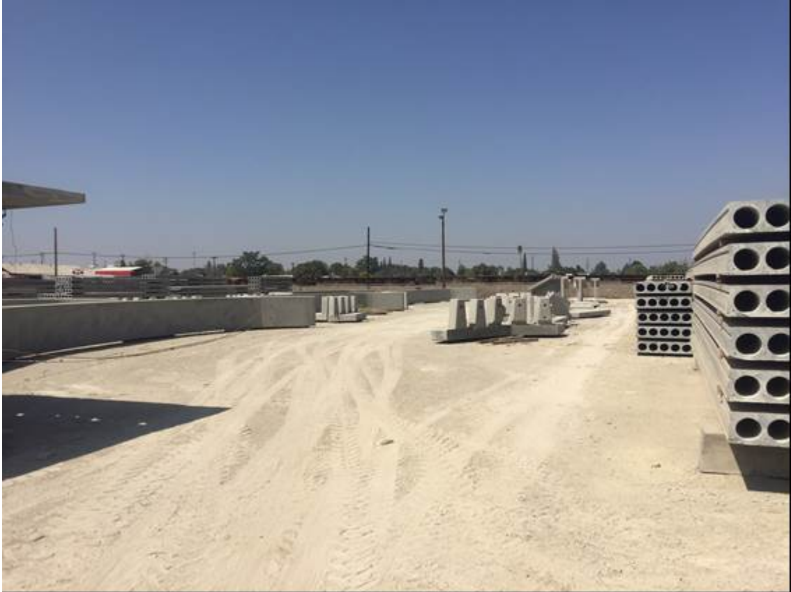
Figure 7: Stored bridge pieces at Bethlehem, Wasco, CA.
