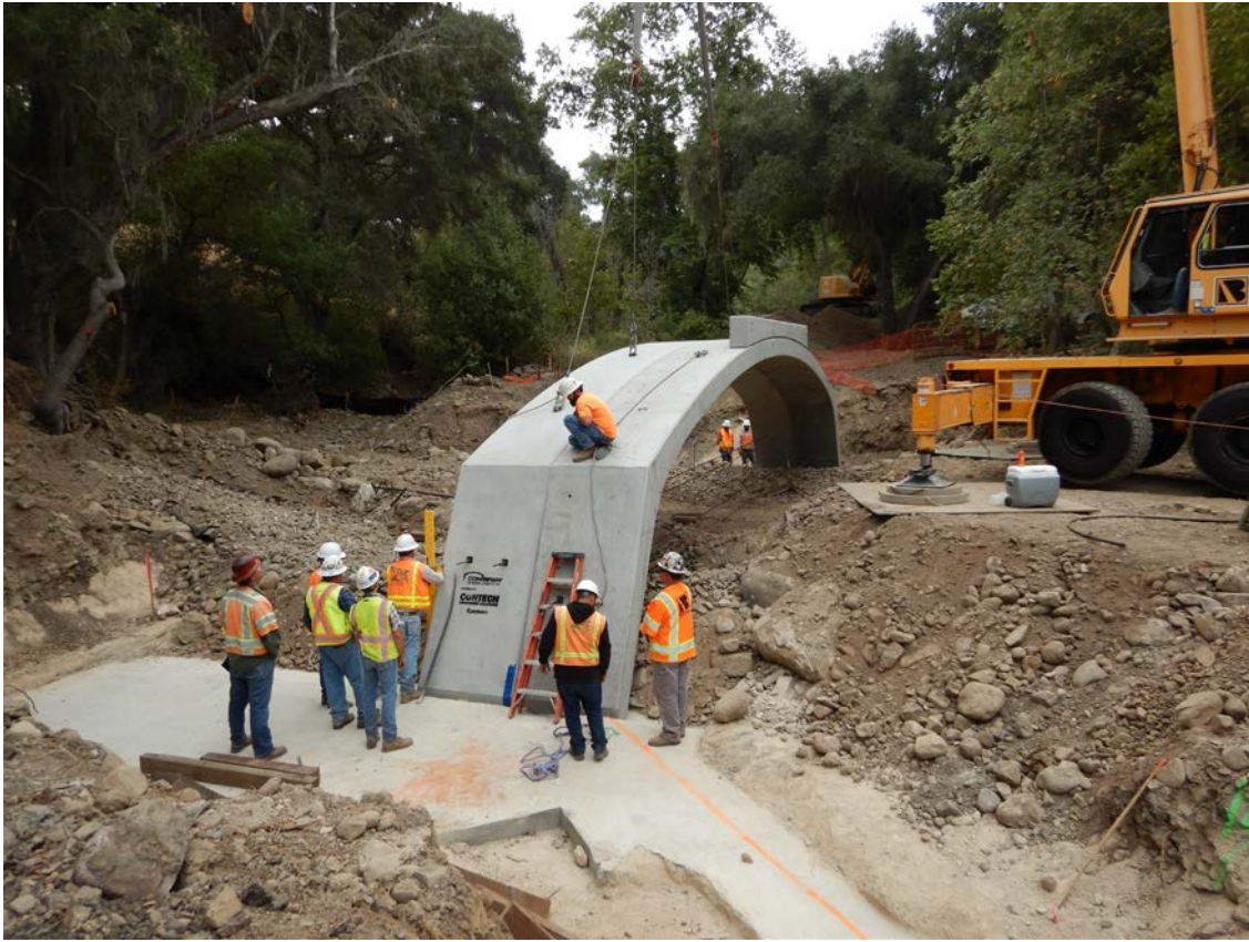
Figure 4: Bridge installation.
