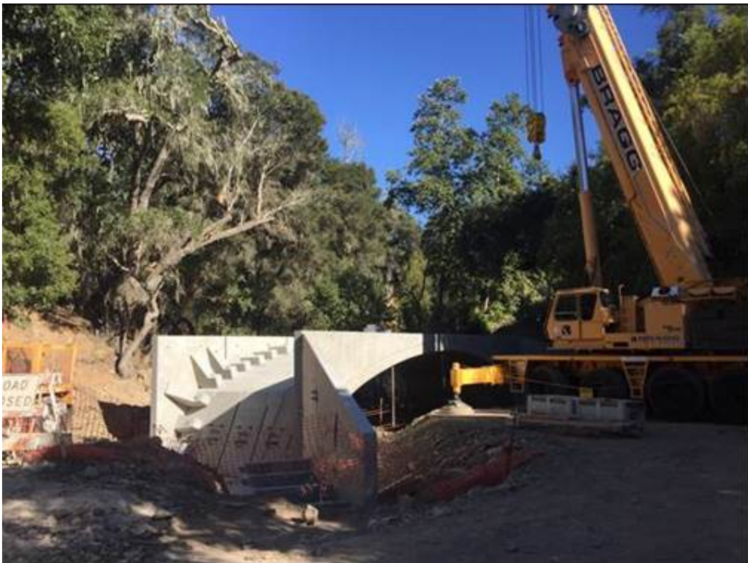
Figure 7: Completed bridge installation on 8/28/18.
