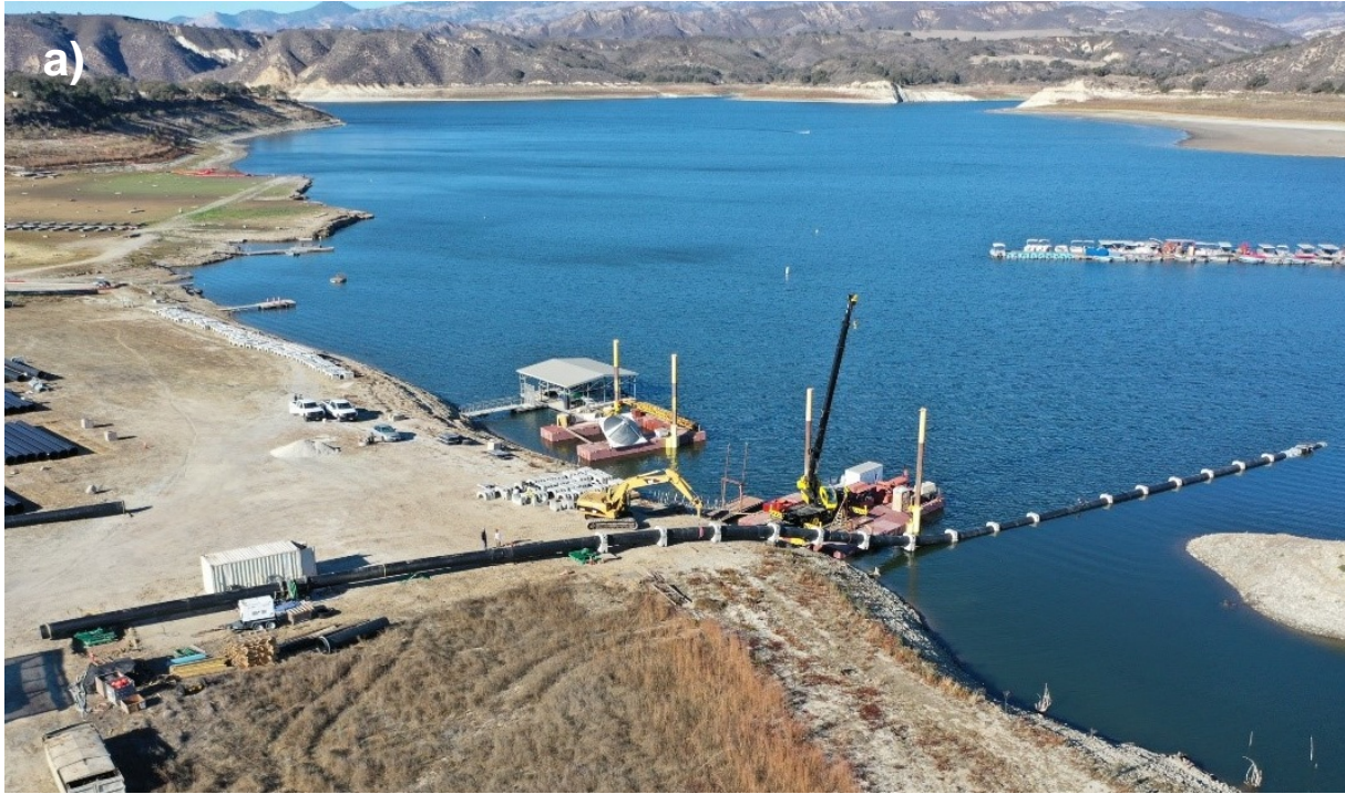
Figure 4: a) HDPE pipeline being fused, concrete weights installed, and being pushed out into the water; b) concrete anchor weights installed on pipeline
