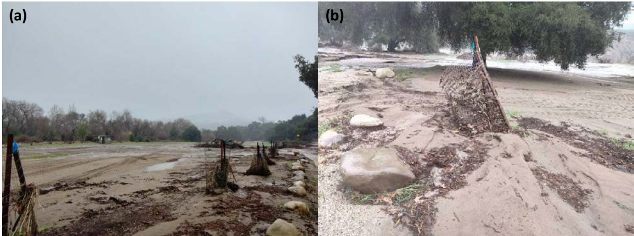
Exhibit 1: Live Oak Camp storm damage showing (a) road approach with inundated trees and (b) a single oak tree pushed over with silt and debris.
