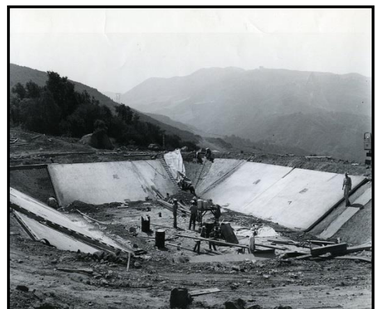
Cachuma Project Construction
