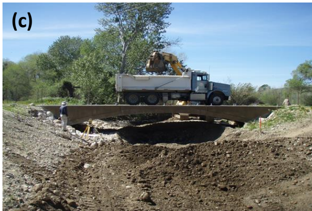
Figure 2: The required fix of the project after strong winter storm flow events specifically the change from the (a) As-Built condition to (b) deposited cobble bar below the bridge, (c) the removal of the cobble bar, and (d) the finished repair returning the project to its design criteria.
