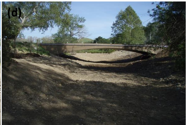
Figure 2: The required fix of the project after strong winter storm flow events specifically the change from the (a) As-Built condition to (b) deposited cobble bar below the bridge, (c) the removal of the cobble bar, and (d) the finished repair returning the project to its design criteria.
