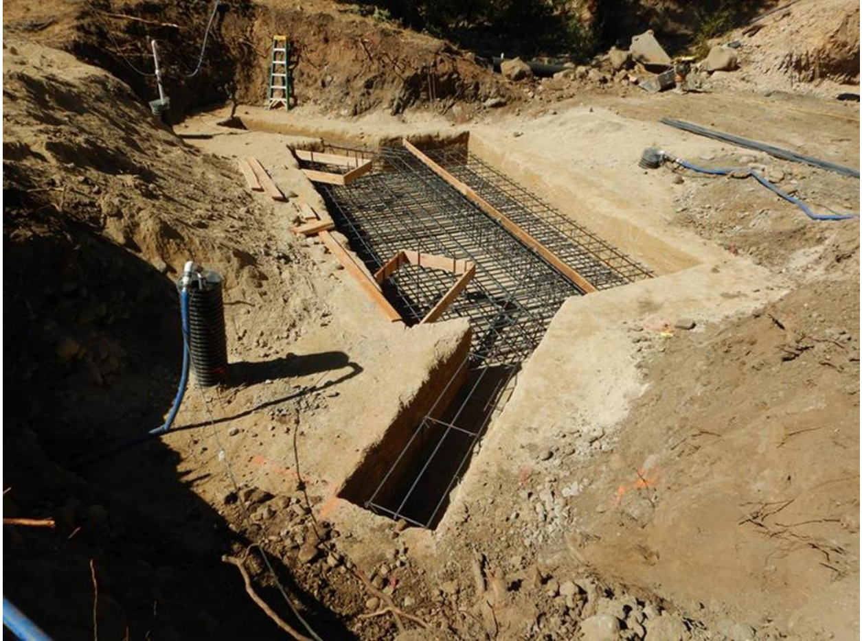
Figure 7: Placing the rebar for the bridge foundation.
