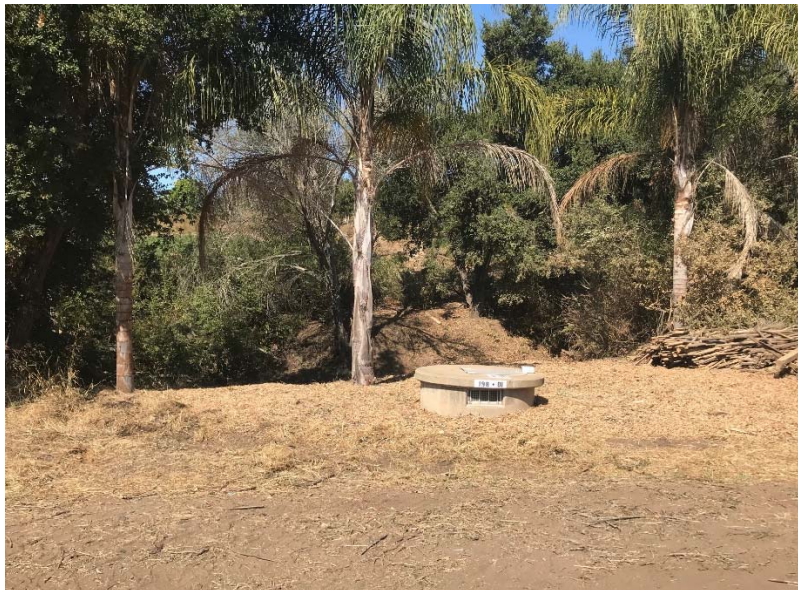
Cleared vegetation around blowoff structure 198+01
