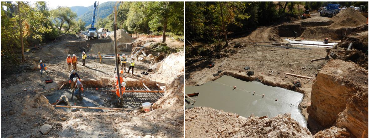
Figure 8: Pouring the bridge foundations.
