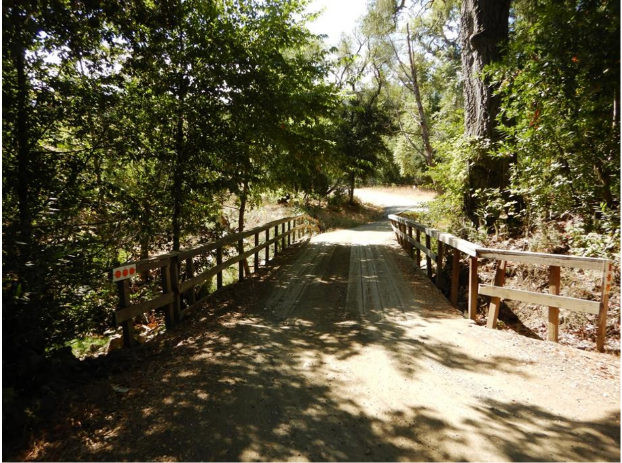
Figure 2: Pre-project conditions looking south across the temporary bridge.
