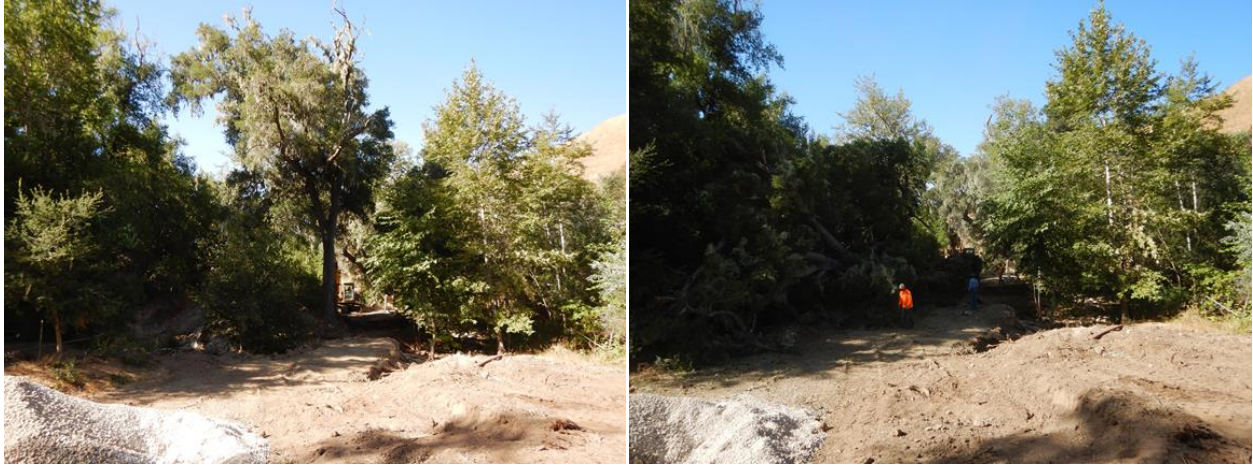
Figure 5: Clearing and grubbing.
