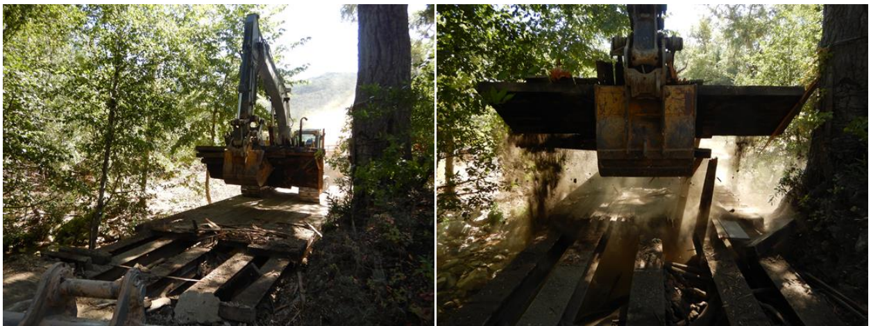
Figure 4: Removal of the temporary bridge.
