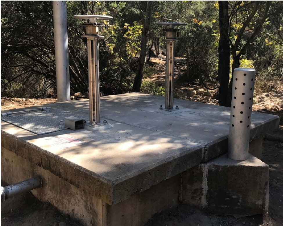
Installed stem extensions and floorstands
