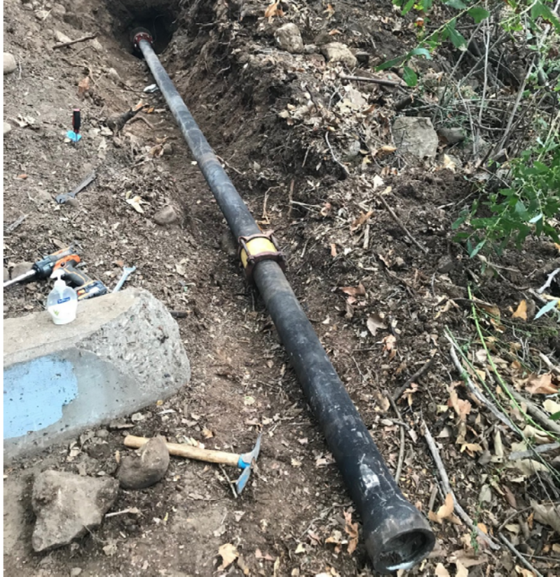
Extension of blowoff piping at structure 477+49
