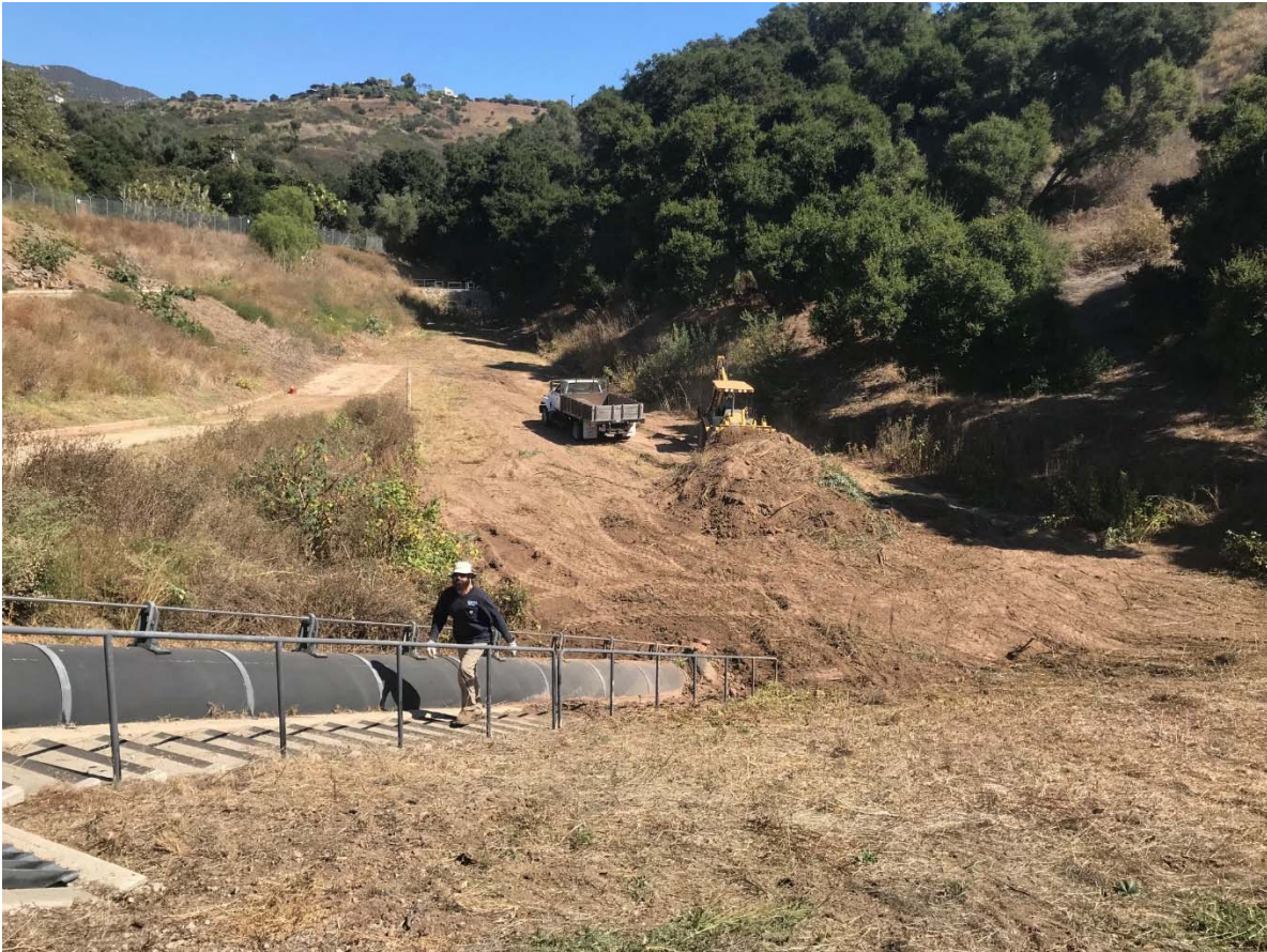
Clearing debris from basin prior to winter storm season
