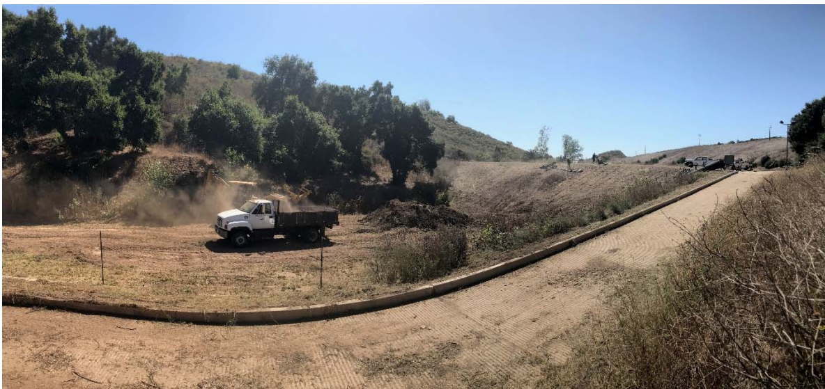
Access route to Lauro Reservoir Debris Basin
