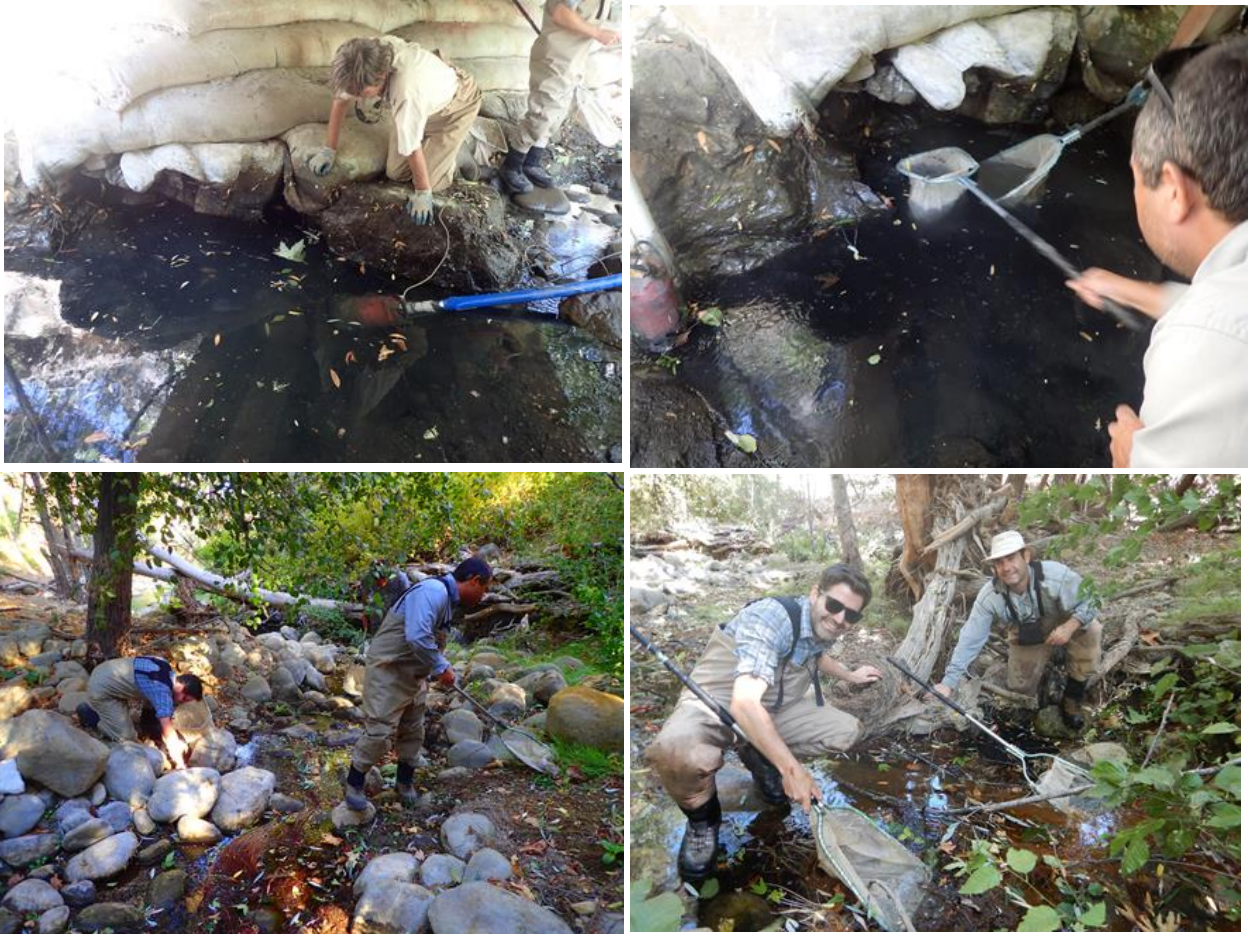
Figure 3: Dewatering the site plus capturing and relocating all aquatic and riparian species.
