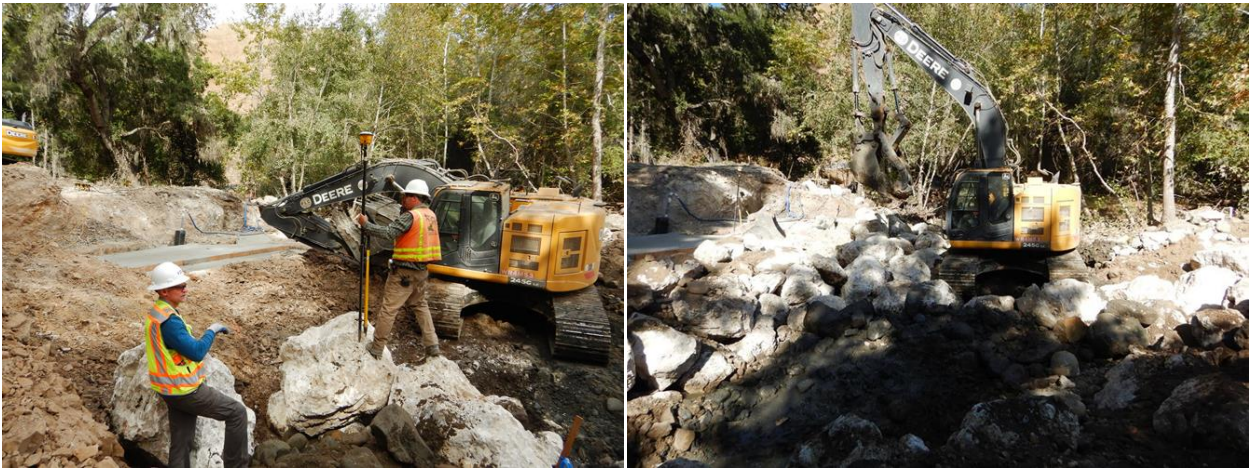
Figure 10: Installing two mid-channel rock weirs.
