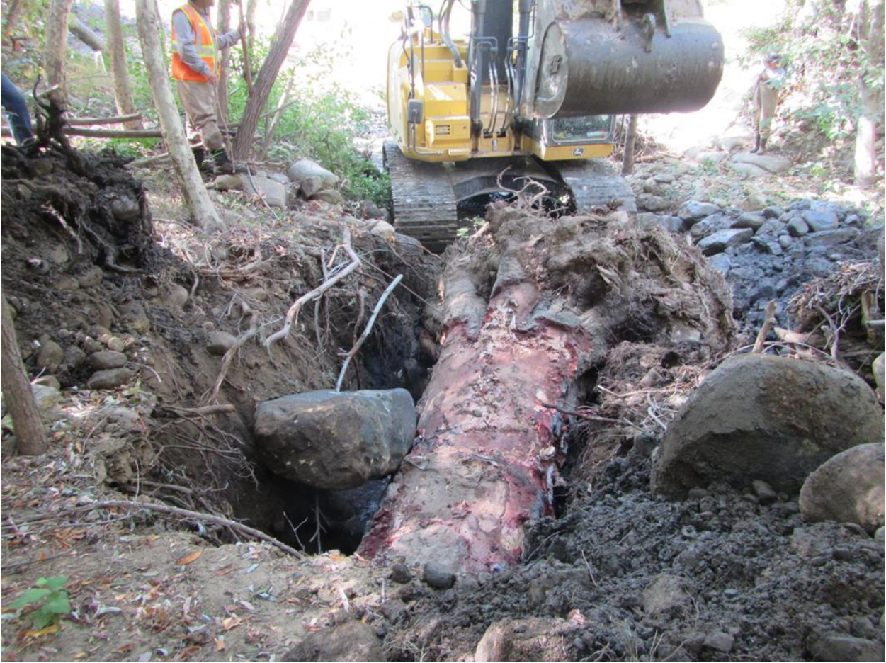
Figure 9: Installing the downstream rootwad.
