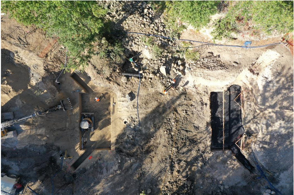
Figure 6: Bridge foundation forming.
