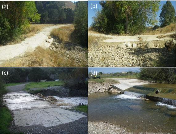
**Figure 1:** Pre-project condition looking (a) across the crossing, (b) upstream at the crossing, and (c+d) the crossing with storm flow.
