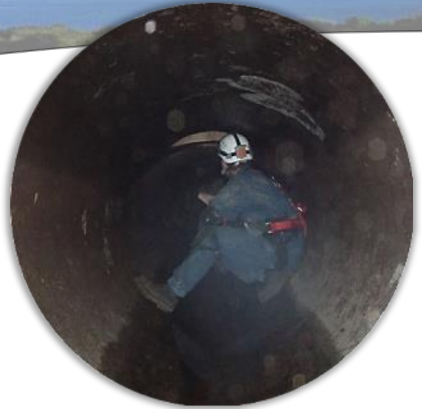
Figure A.13 Previous Inspection of SCC Interior
