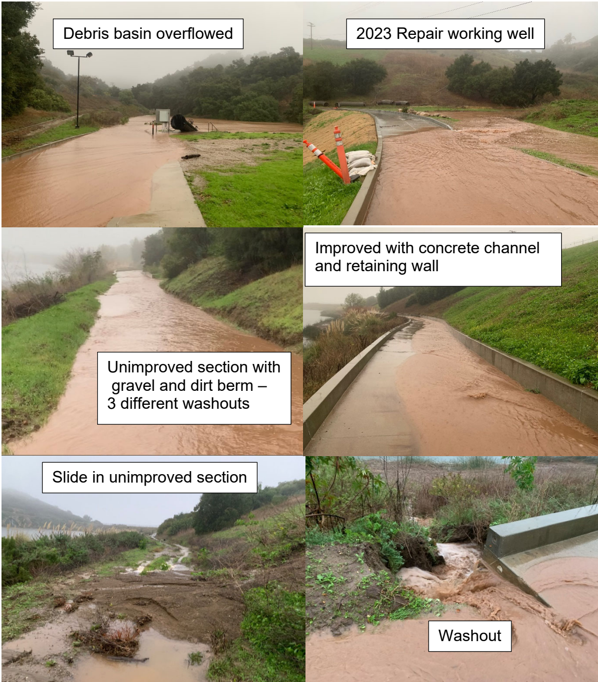
Lauro Reservoir Bypass Channel Road on February 4 th , 2024
