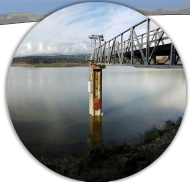
Figure A.7 North Portal Intake Tower
