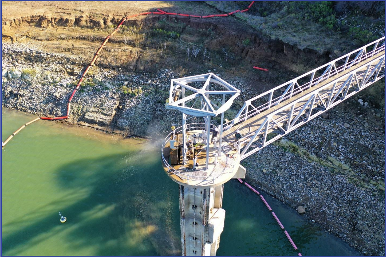
Figure 2. Lake Cachuma North Portal Intake Tower Maintenance
