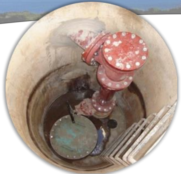
Figure A.4 Inside of Blow Off Structure
