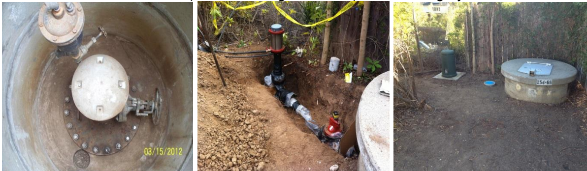
AVAR 254+66 Rehabilitation (Before, During, and After) USBR Category 1 Recommendation
