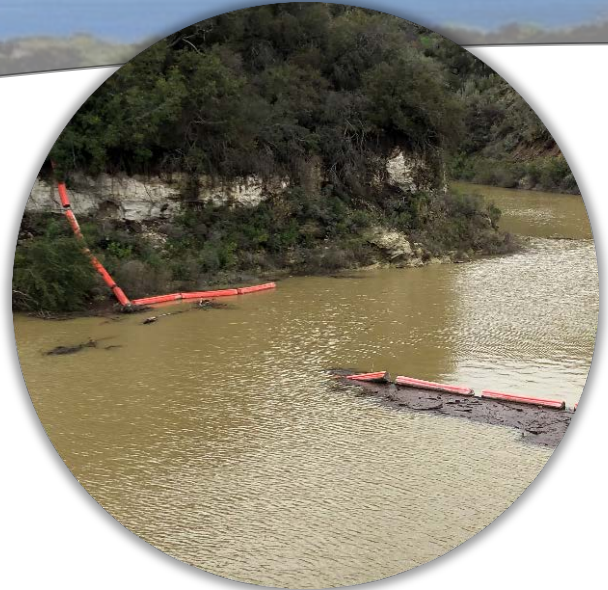
Figure A.16 Log Boom Shackle Failure
