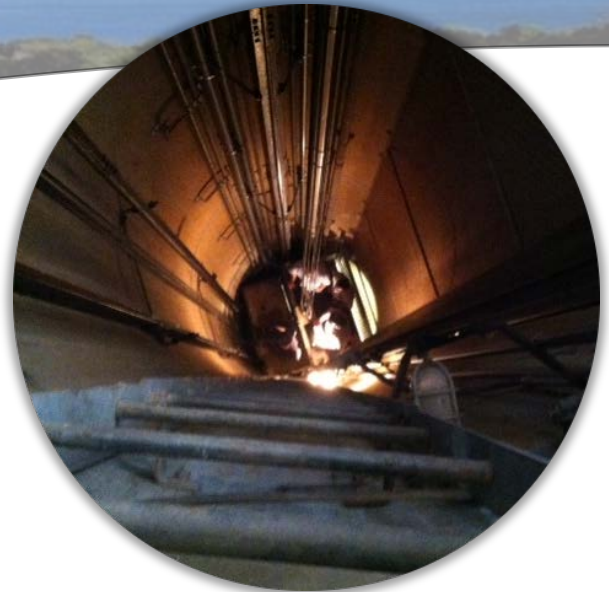
Figure A.2 North Portal Elevator Shaft
