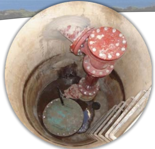
Figure A.4 Inside of Blow Off Structure
