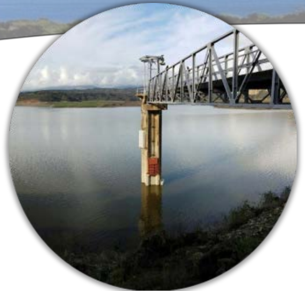
Figure A.7 North Portal Intake Tower
