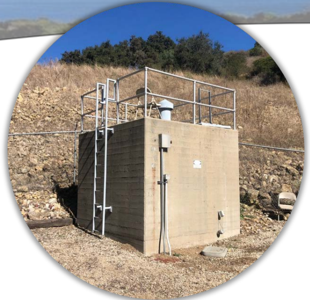
Figure A.1 Lauro Outlet Works Tunnel Access House
