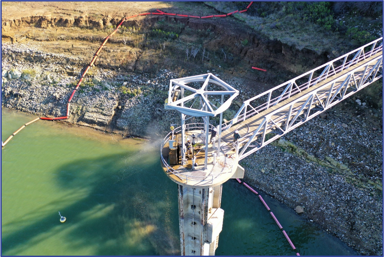
Figure 2. Lake Cachuma North Portal Intake Tower Maintenance
