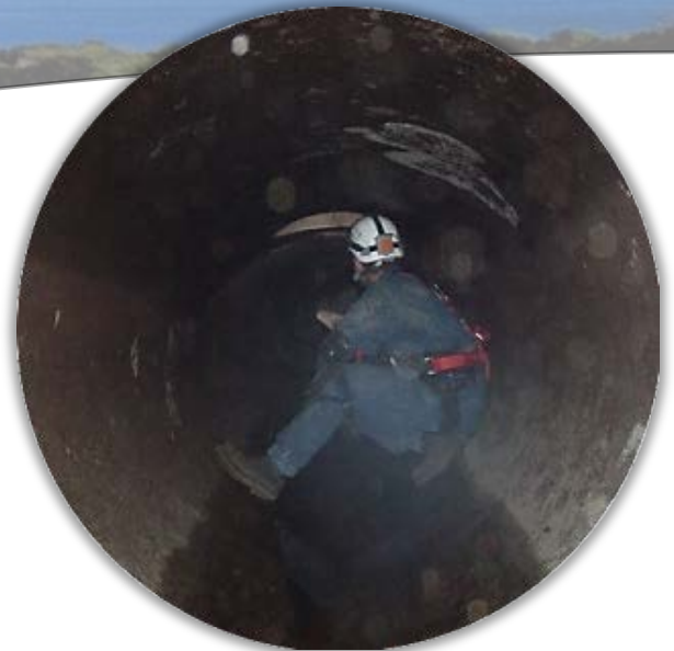
Figure A.13 Previous Inspection of SCC Interior
