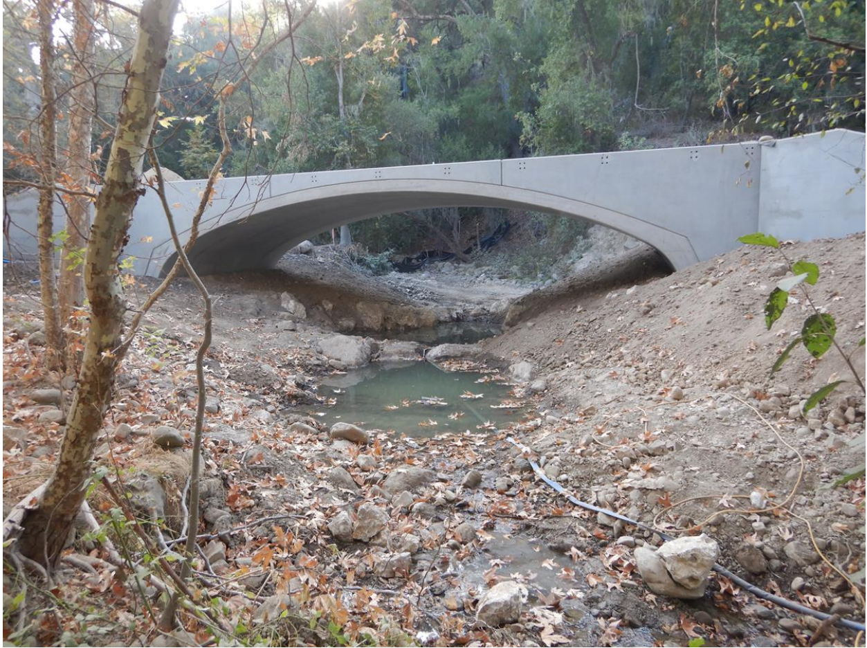
Figure 10: Stream bottom with two created step pools looking upstream under the bridge.
