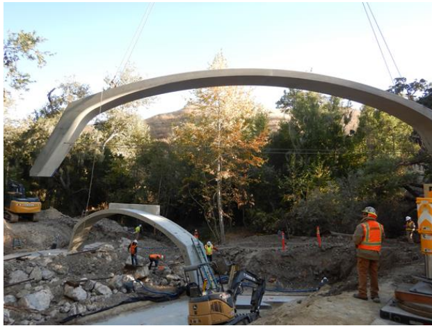
Figure 4: Bridge install.
