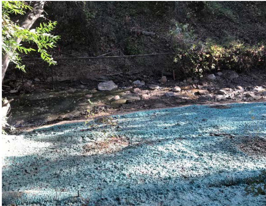
San Jose Creek crossing post-project with native hydro-seeding and tree planting and invasive Arundo removed
