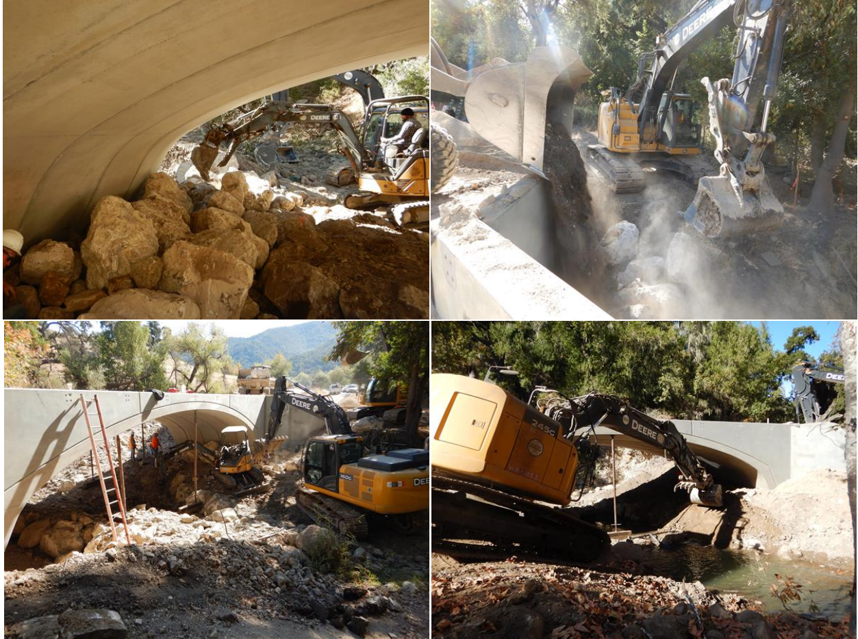
Figure 9: Installing rock slope protection and finalizing the stream channel.
