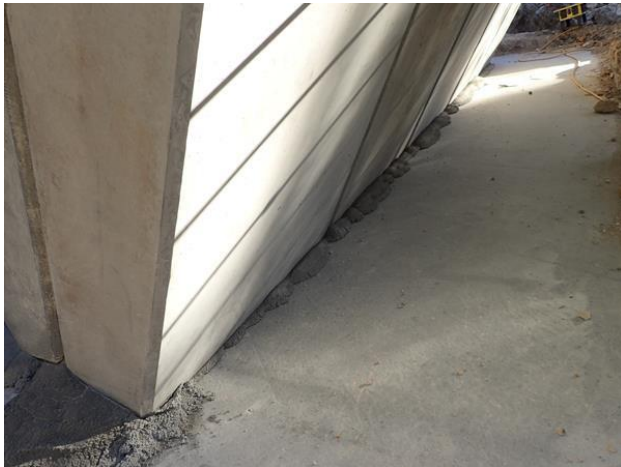
Figure 7: Placing grout under the arches and wing walls.
