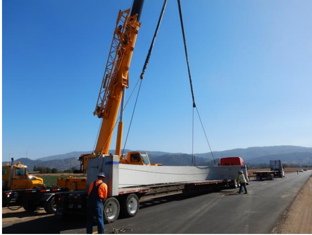
Figure 6: Arch piece transfer from low to high trailer.
