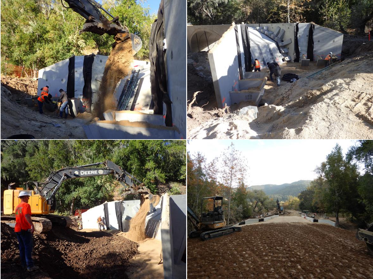
Figure 8: Backfilling of the bridge.
