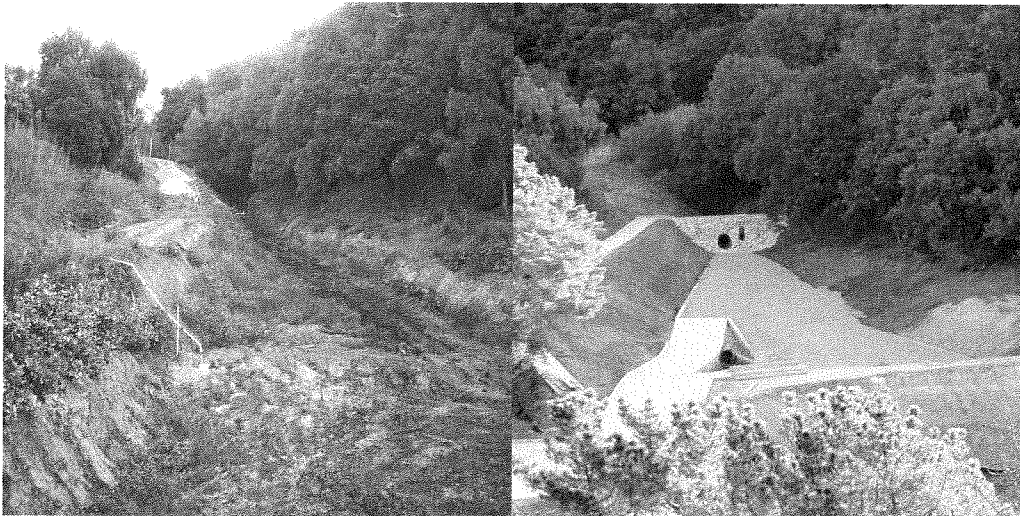
Picture 1 –Lauro Retention Basin Overview Pre-Construction
