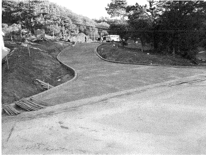
Picture 2 –Concrete Access Rd 1/16/09
