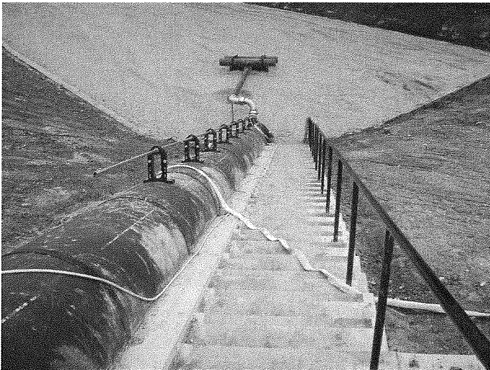
Picture 4 – Decant Structure 1/10/09
