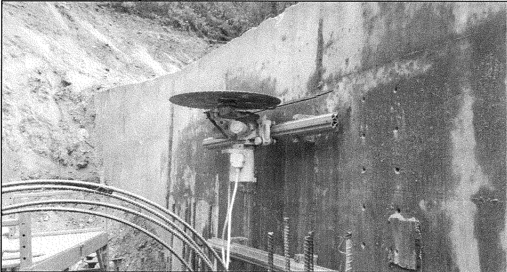
Cutting concrete for penetration into existing structure
