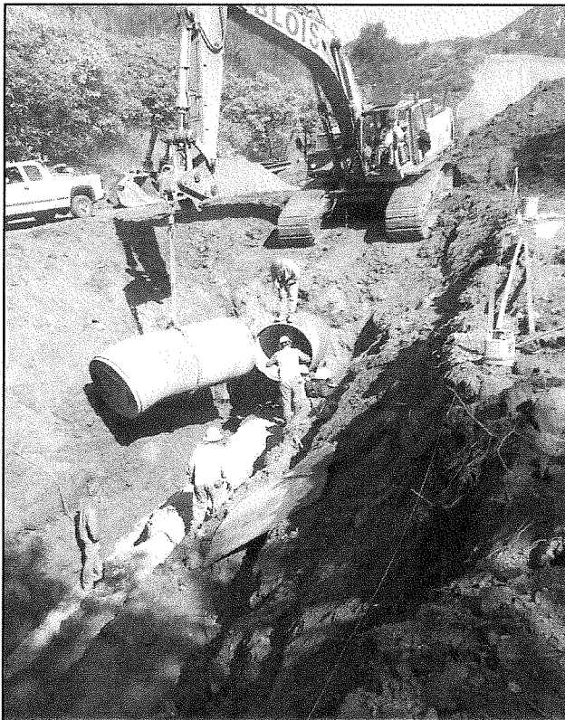
Setting pipe into place
