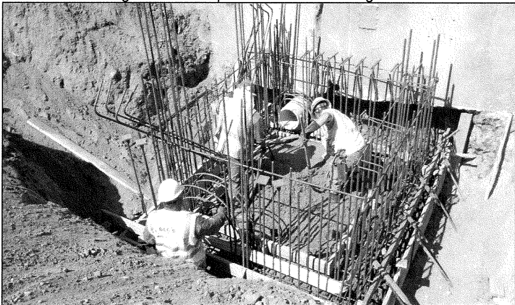
Placing concrete base for Junction Structure modifications
