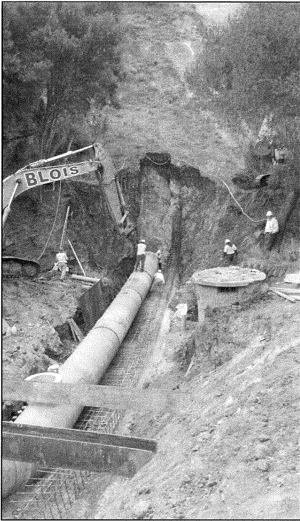
Pipe being laid across creek
