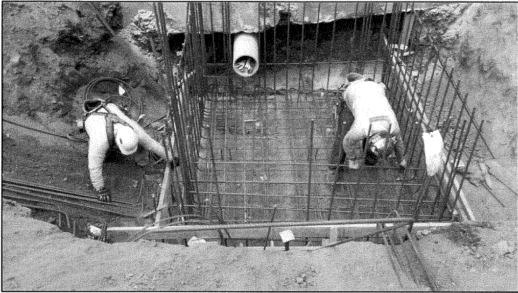
Placing steel for Junction Structure Modifications
