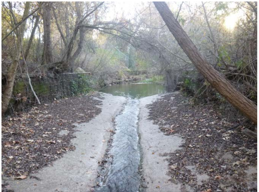
Figure 7: Maria Ygnacio Creek at San Marcos Road showing the fish passage impediment where the SCC crosses the creek with protective concrete on top.
