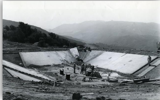
Construction of Bradbury Dam
