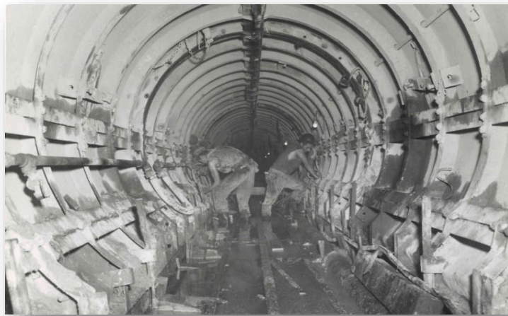
Tecolote Tunnel Construction
