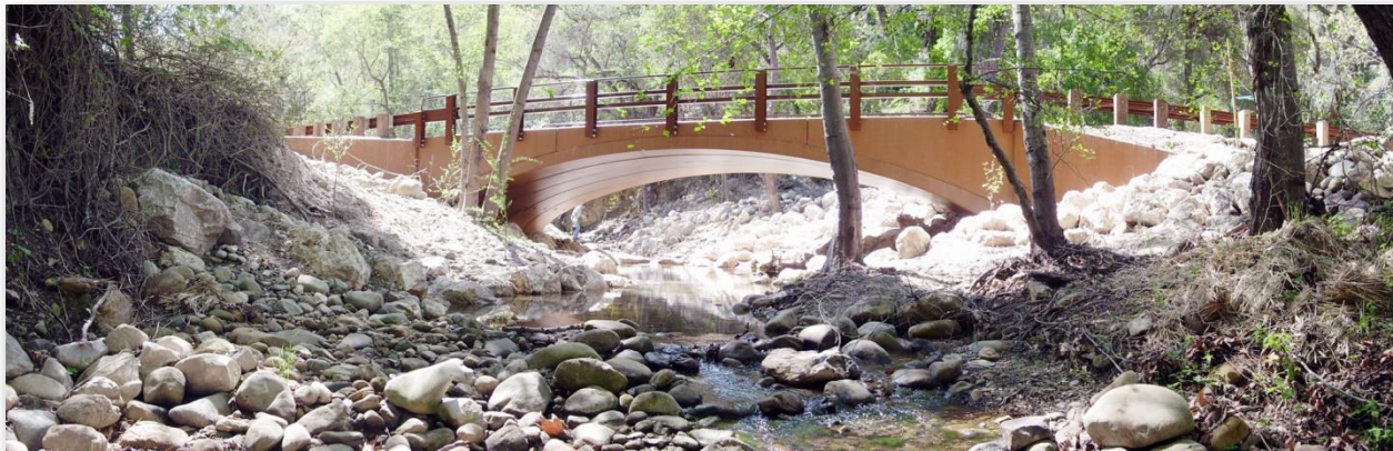
Quiota Creek Fish Passage Project
