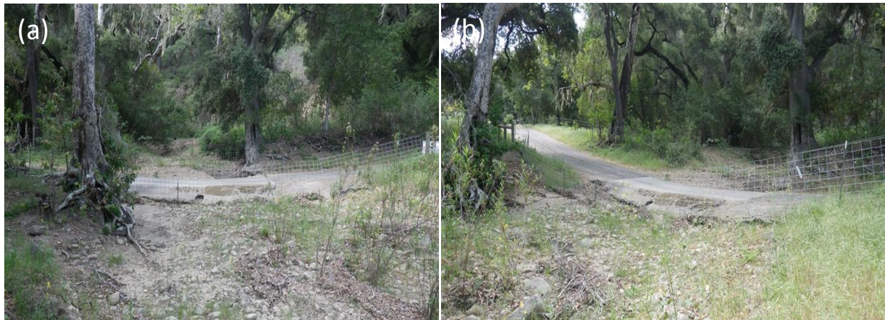
Figure 1: Pre-project condition looking (a+b) upstream over the crossing.
