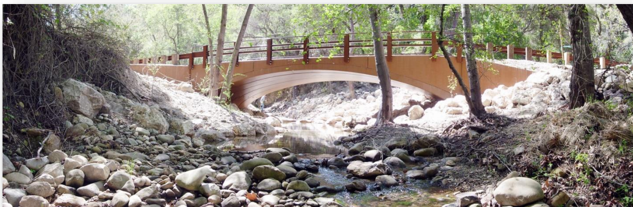
Quiota Creek Fish Passage Project
