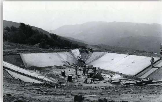
Construction of Bradbury Dam
