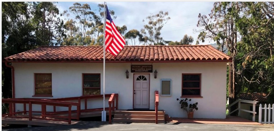
Cachuma Operation and Maintenance Board Meeting Room
