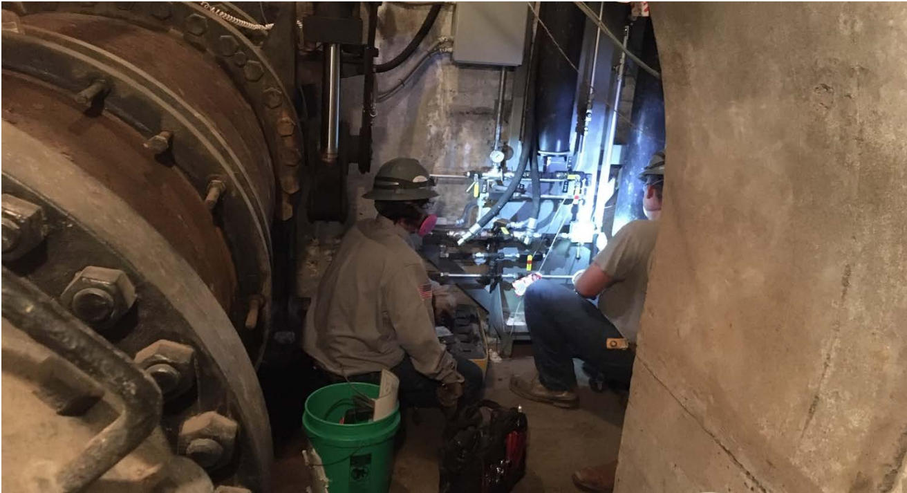
Lauro Hydraulic Solenoid Valve Replacement
