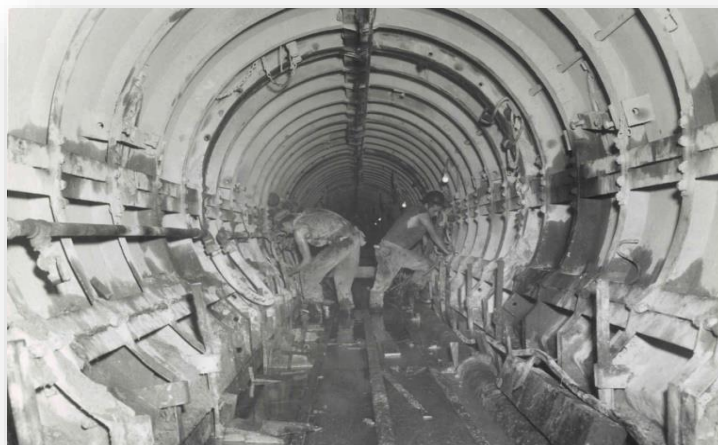
Tecolote Tunnel Construction
