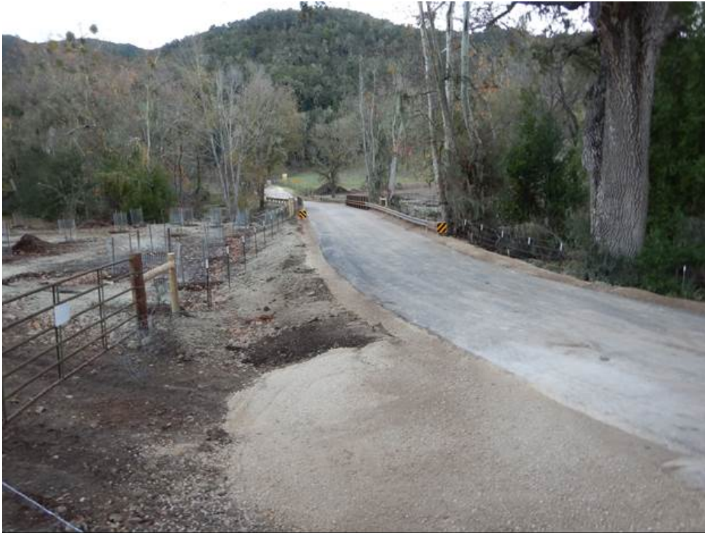
Figure 5: Completed bridge rails and guardrails.
