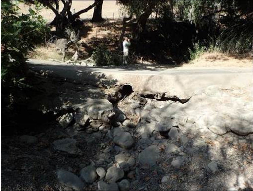
Figure 1: Pre-project condition looking upstream.
