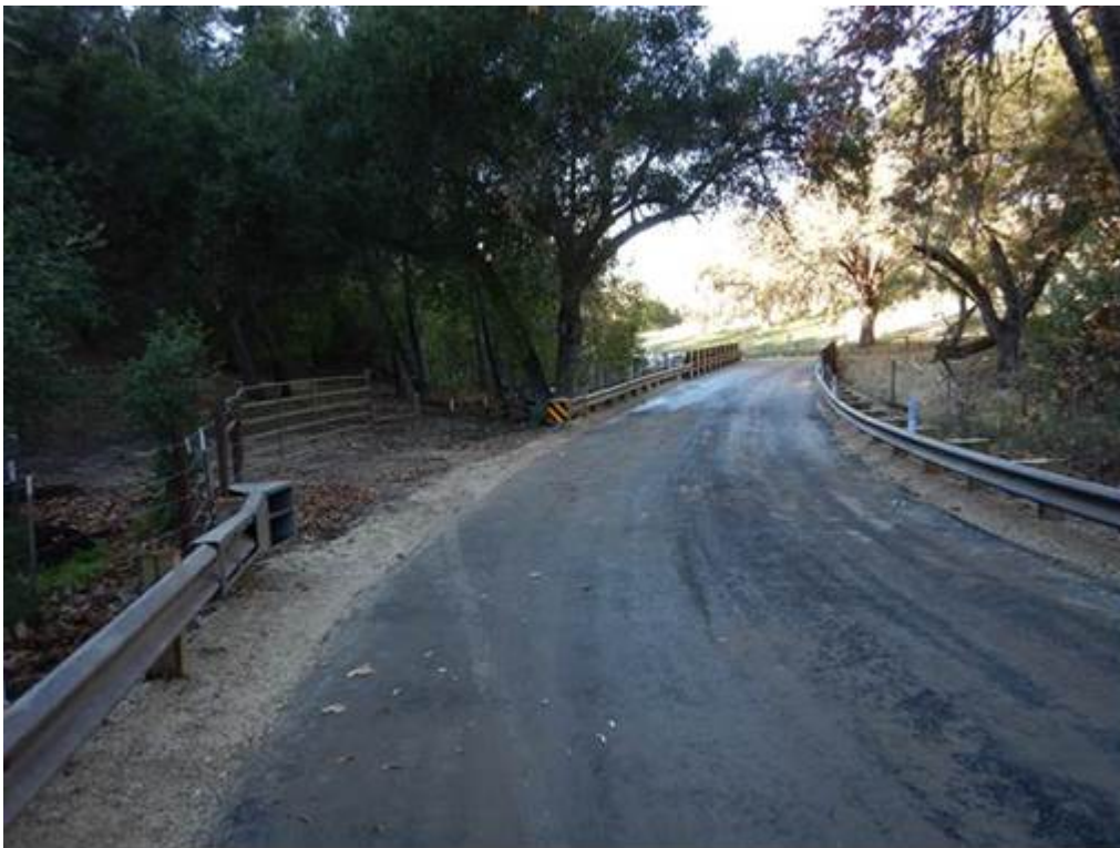
Figure 2: Completed paving and guardrail and bridge rail installed.
