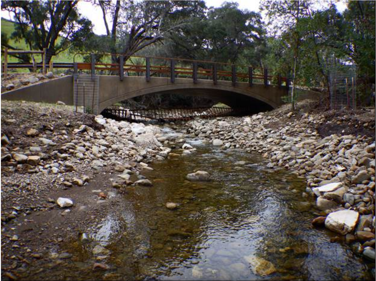
Figure 7: The project after winter stormflow events (3/1/19).
