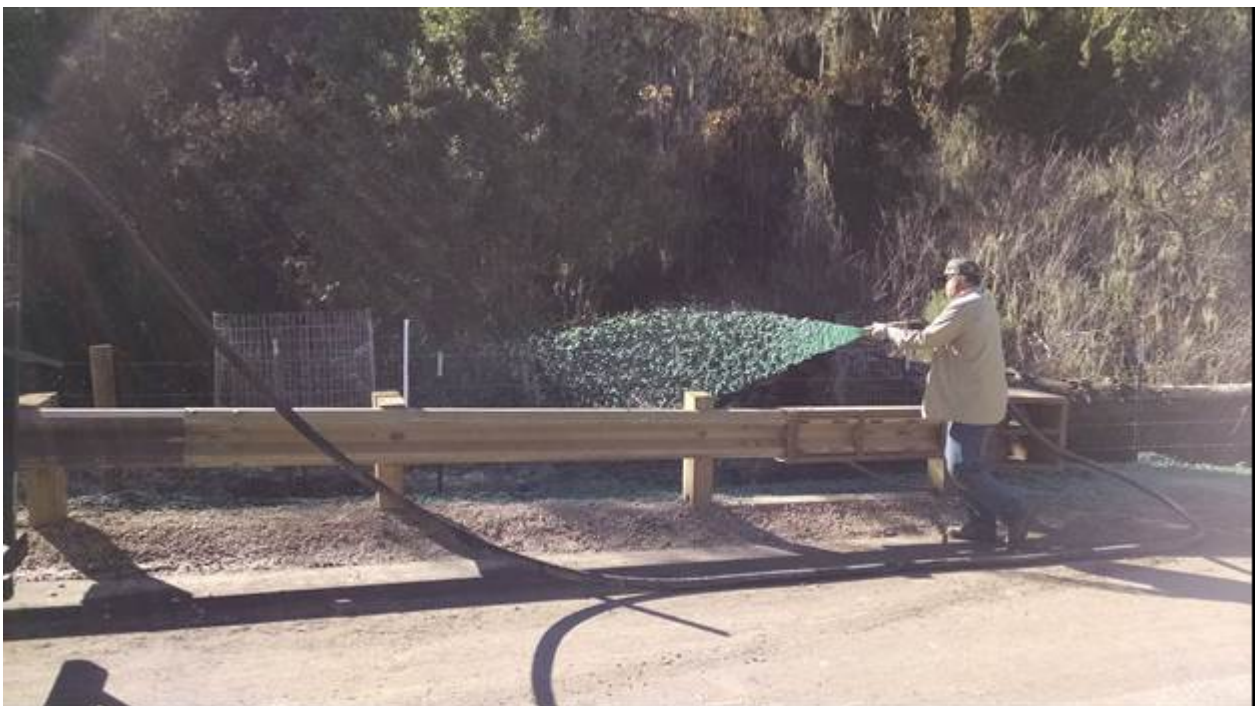
Figure 4: Hydro-mulching/seeding the project site.
