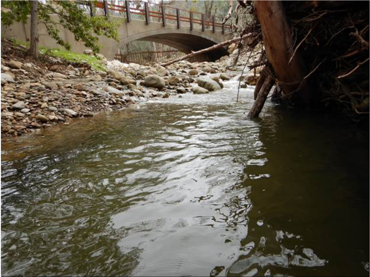
Figure 7: Project after winter stormflow events.
