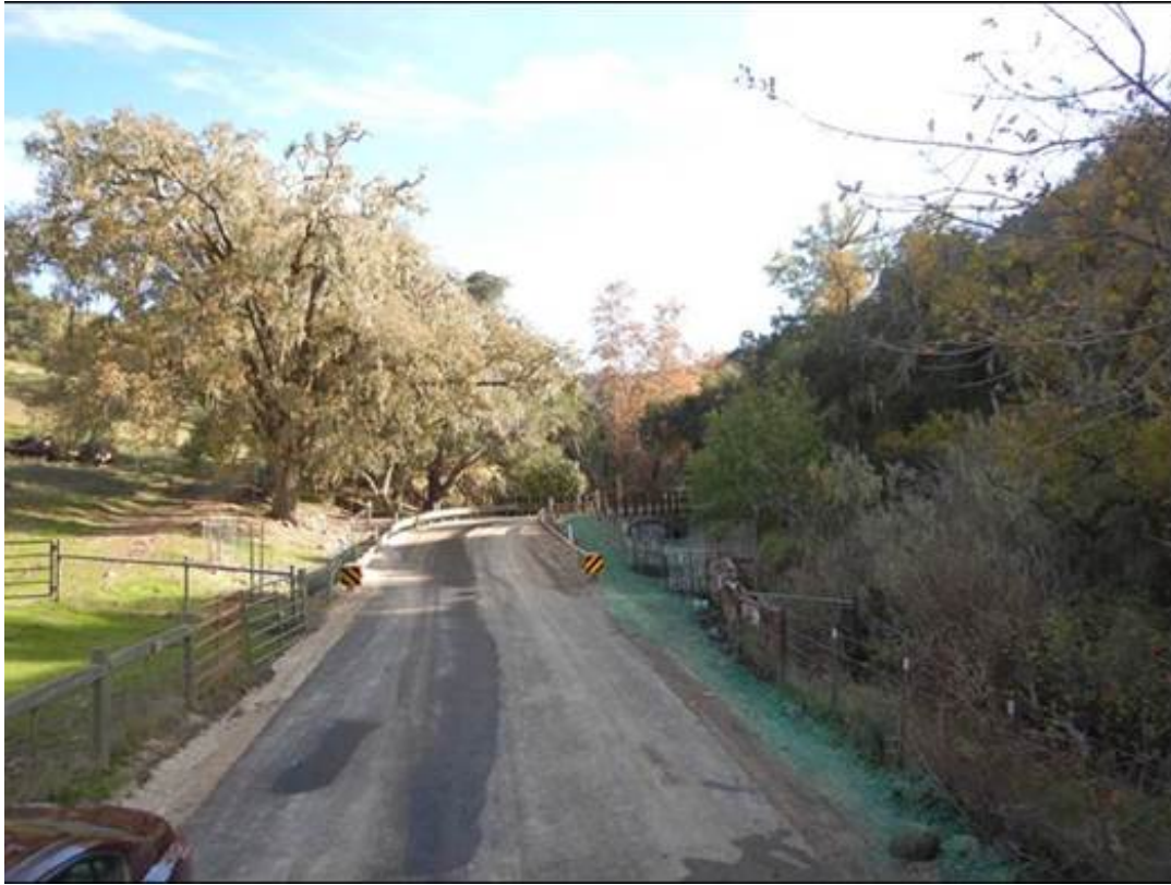
Figure 5: Completed hydro-mulching and seeding.
