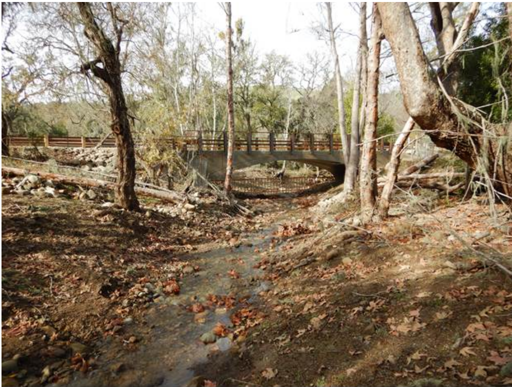
Figure 6: Completed project with the first streamflow event of the year.
