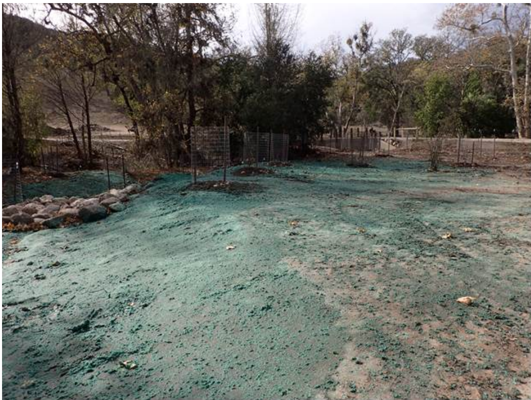
Figure 4: Hydro-mulching/seeding of the project site.
