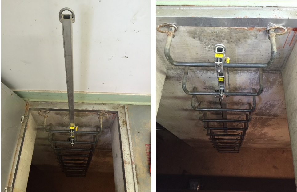
New ladder extension
