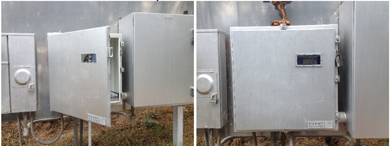
Boundary meter window installation
