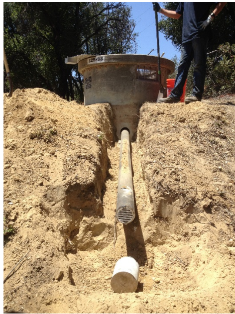
AVAR drain installation
