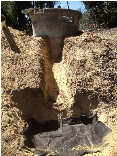
AVAR drain installation
