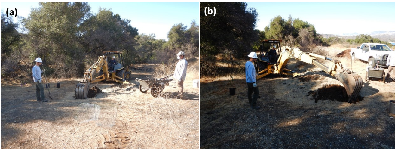
Figure 19: Digging tree holes with the backhoe for planting.
