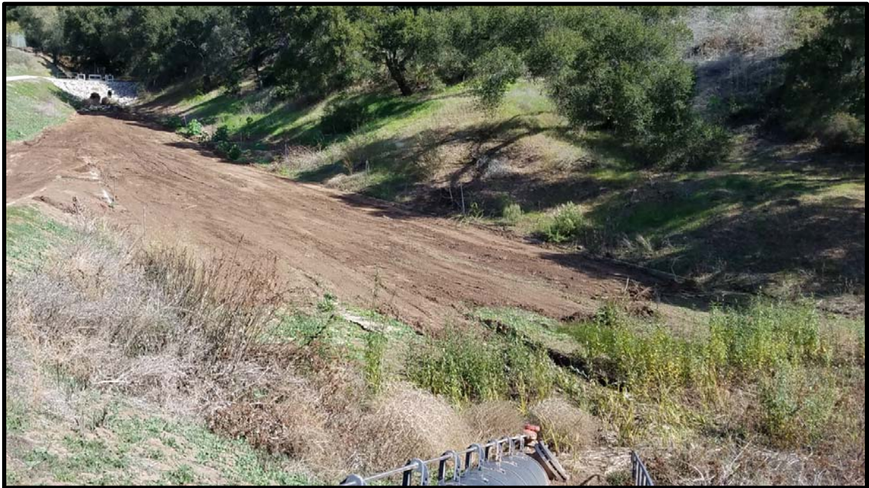
Debris Basin Maintenance
